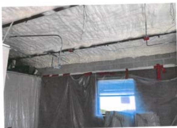
New Ceiling Insulation
