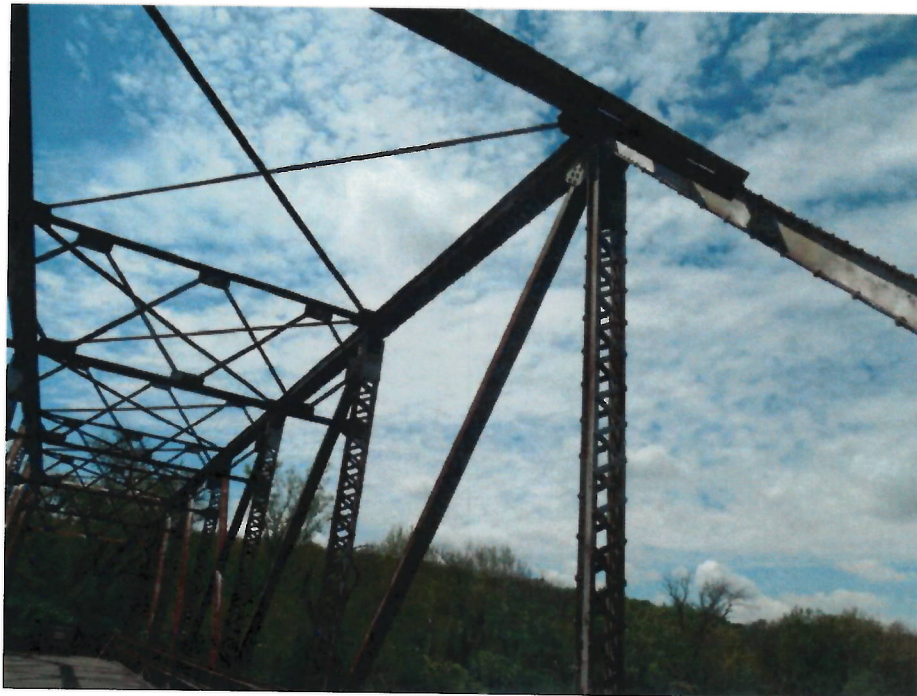
Photo 12 - Top of Center Truss - South
