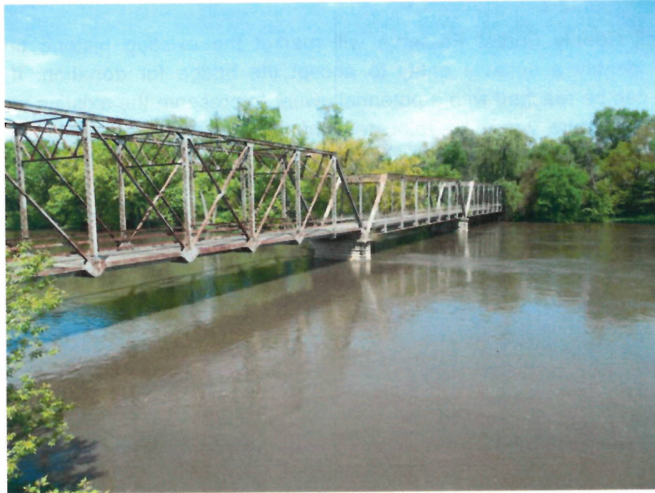
Photo 1 - Looking East at downstream face of bridge
