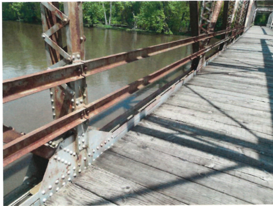
Photo 5 - Railing on North Side of West Truss
