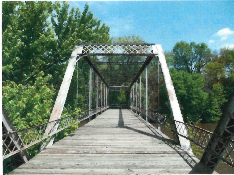
Photo 13 - Looking East thru East Truss
