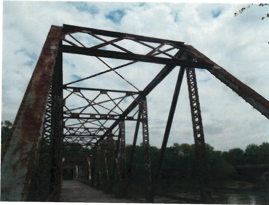
Photo 3 - Looking east thru truss from west end of bridge
