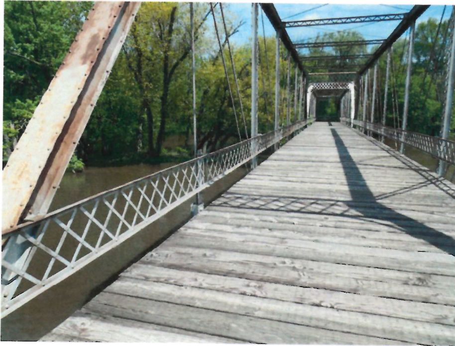
Photo 11 - Looking East thru Center Truss at Railing and Timber Deck
