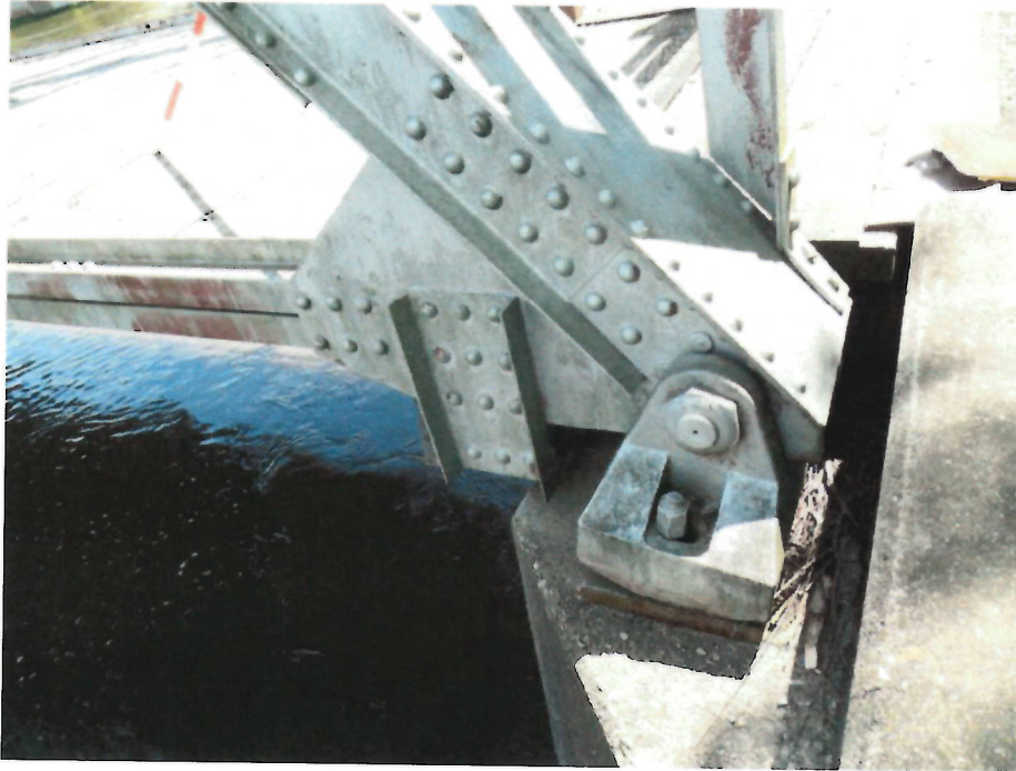
Photo 7 - Northwest Bearing at Abutment
