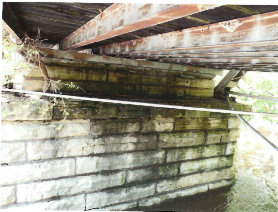
Photo 15 - East face of East pier and underside of deck
