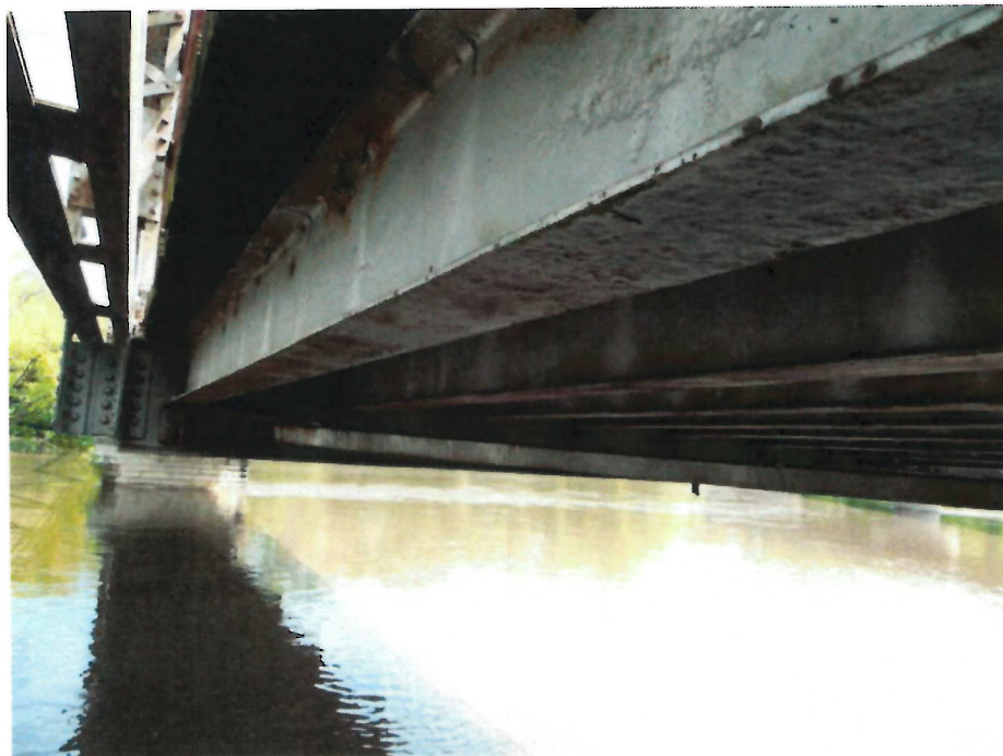
Photo 6 - Looking East at Beams under West Truss
