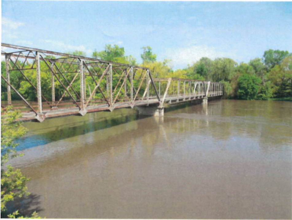
Photo 1 - Looking East across South Bridge Fascia
