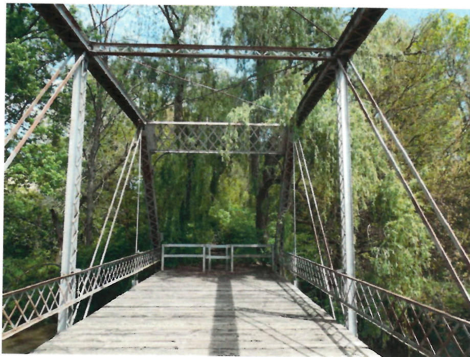
Photo 16 - Looking at East End of Bridge
