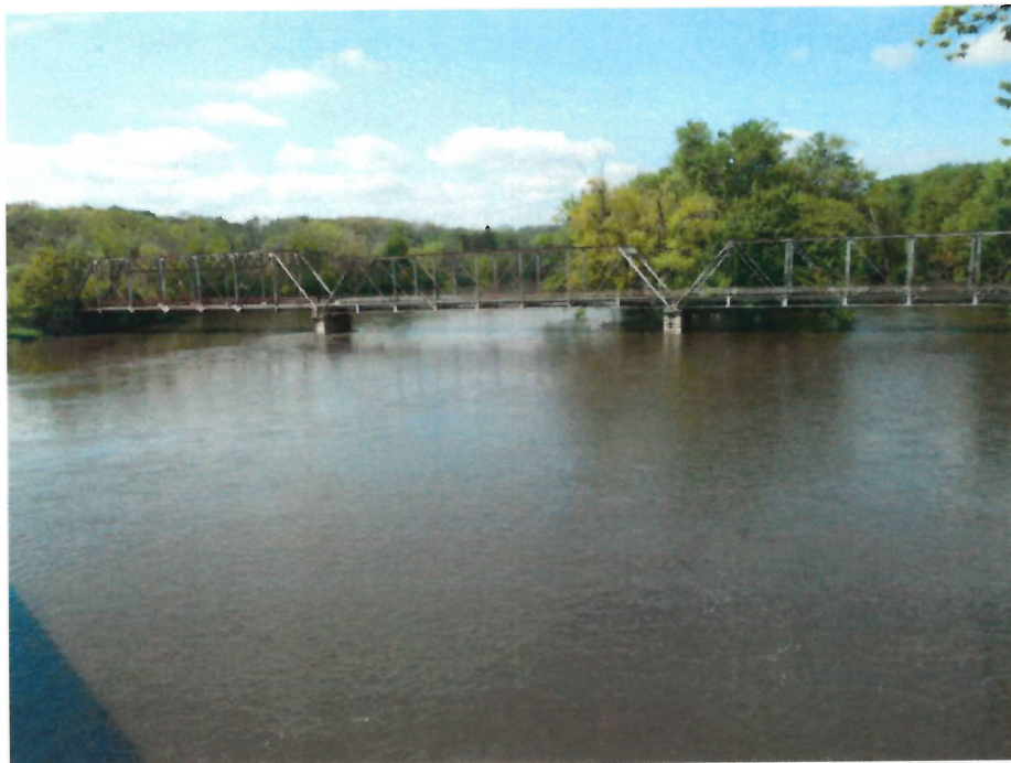
Photo 2 - Looking west at downstream face of bridge
