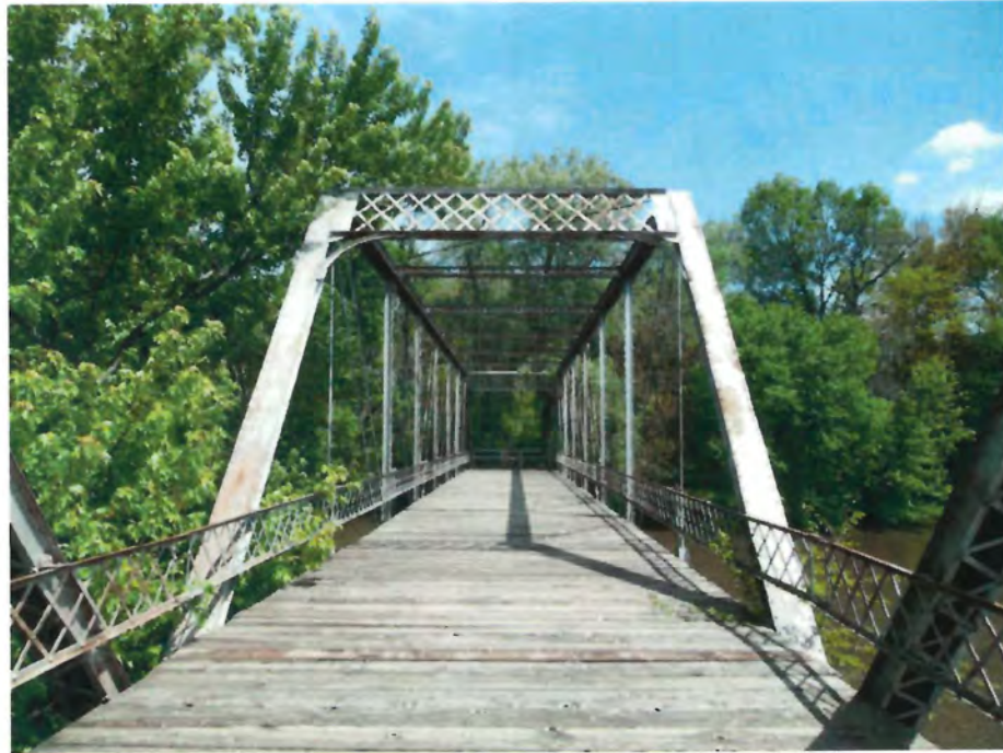
Photo 13 - Looking East thru East Truss
