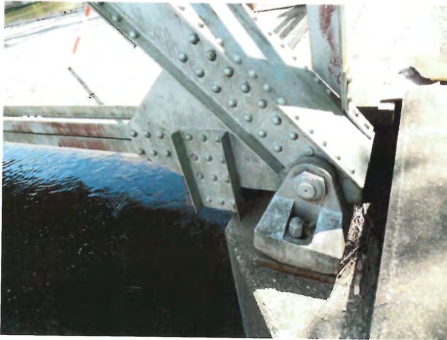
Photo 7 - Northwest Bearing at Abutment
