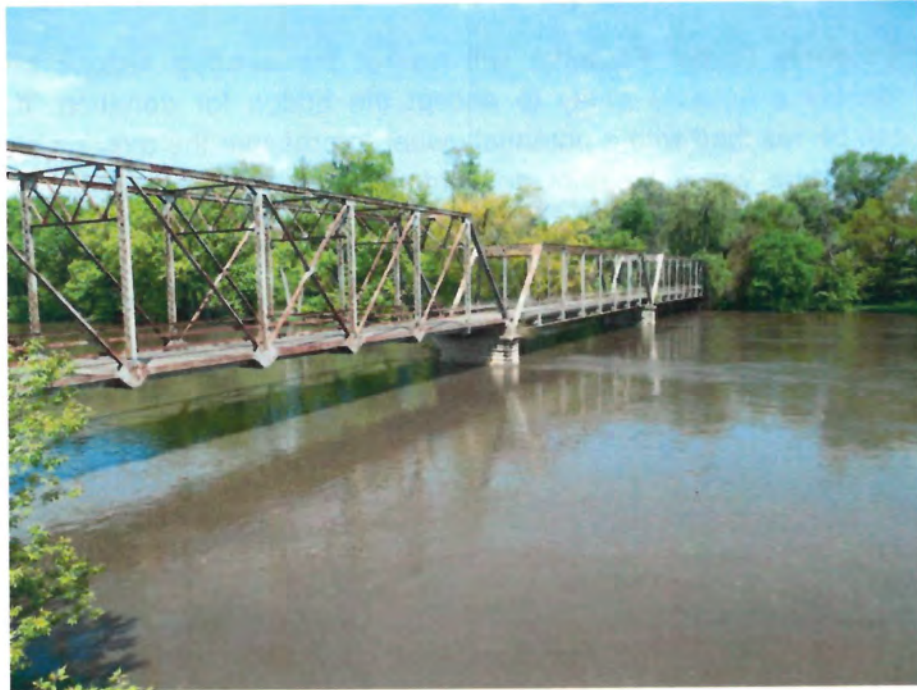
Photo 1 - Looking East at downstream face of bridge
