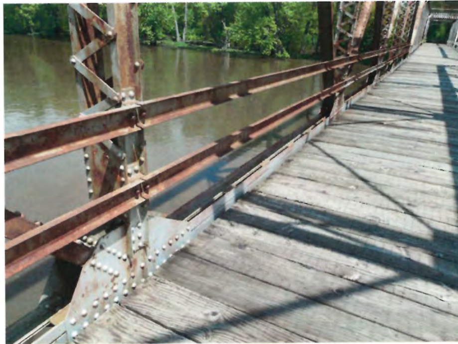
Photo 5 - Railing on North Side of West Truss
