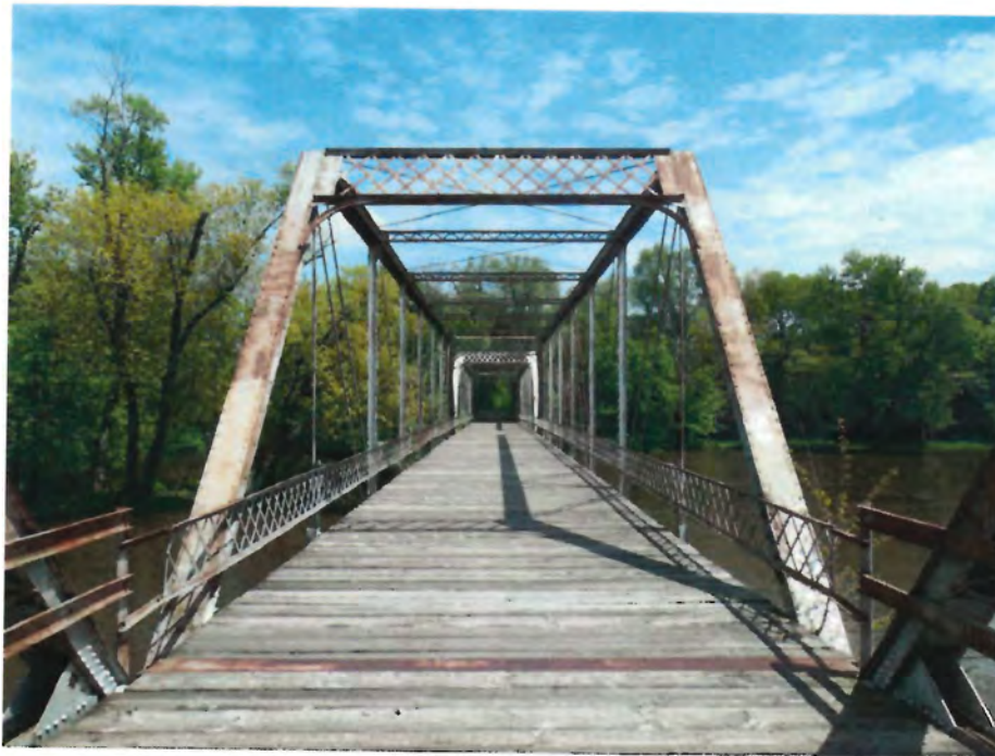
Photo 8 - Looking East thru Center Truss
