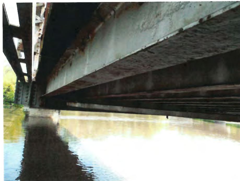
Photo 6 - Looking East at Beams under West Truss
