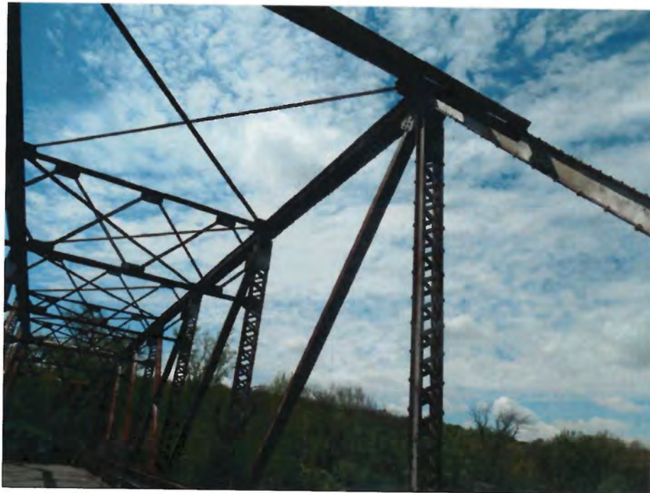
Photo 12 - Top of Center Truss - South
