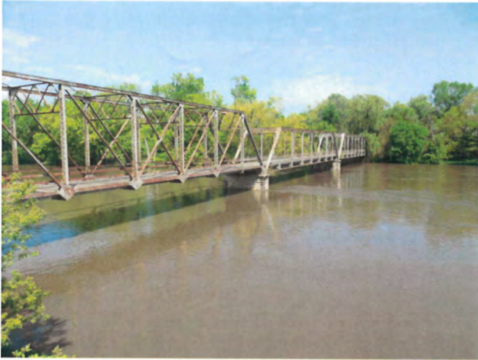
Photo 1 - Looking East across South Bridge Fascia
