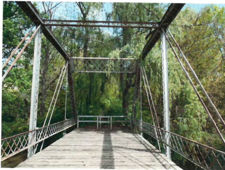
Photo 16 - Looking at East End of Bridge
