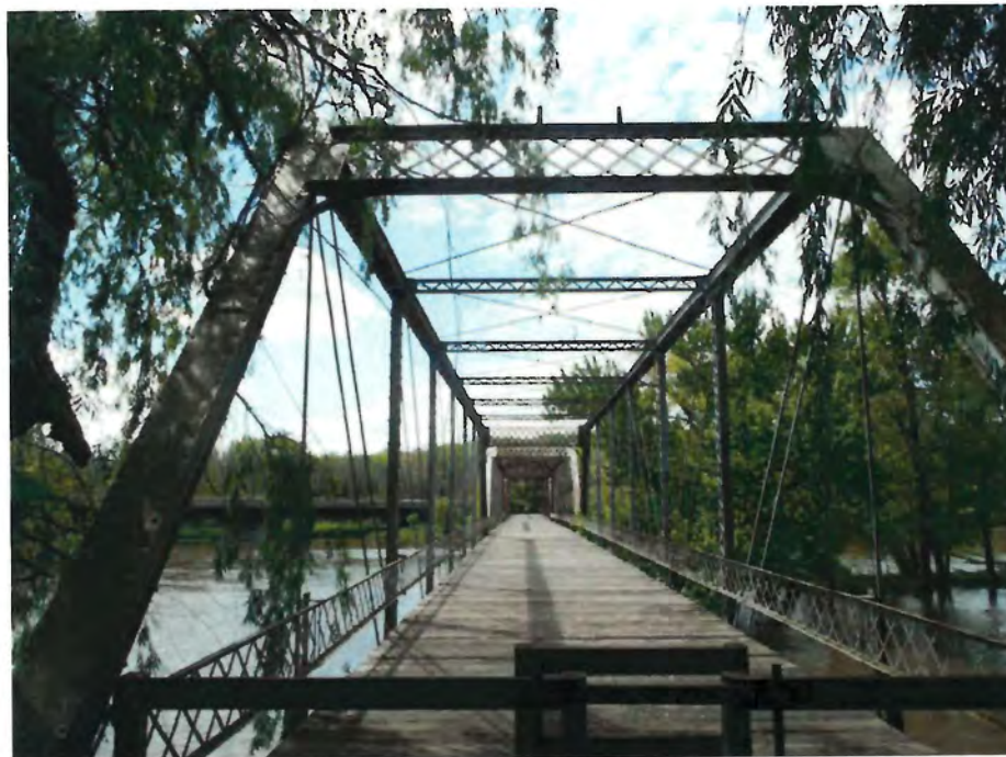
Photo 18 - Looking West from East end of bridge
