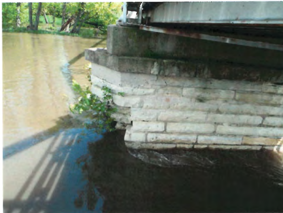
Photo 10 - Northwest Side of West Pier
