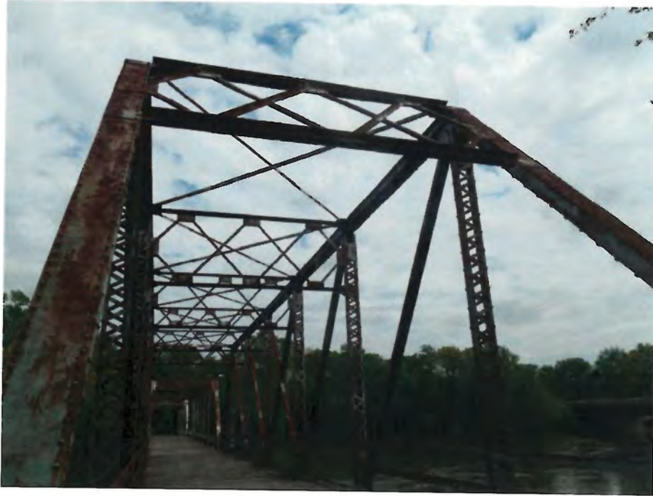
Photo 3 - Looking east thru truss from west end of bridge
