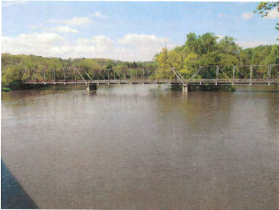
Photo 2 - Looking West across South Bridge Fascia
