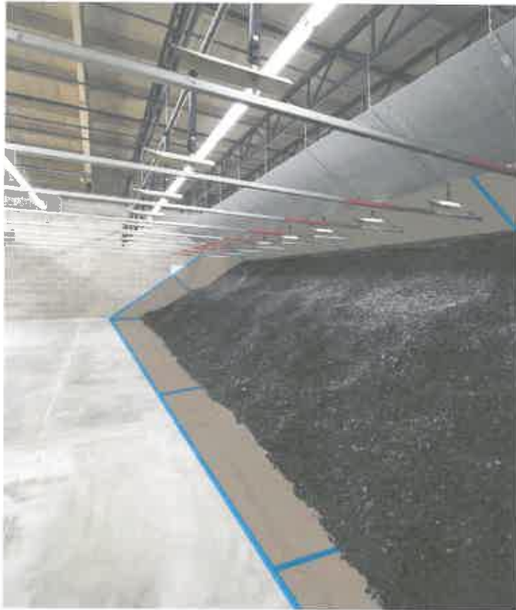
FIGURE 3. PROTECT SURROUNDING SURFACES BEFORE APPLYING FIRE RETARDANT
