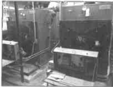
Non-Condensing Boilers
