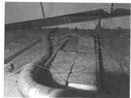
Insulation Over Office Space
