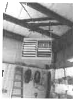
Typical Unit Heater
