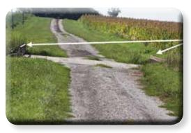
Here's another narrow, poor condition road with no shoulders and a narrow, **unmarked bridge,** which could be very dangerous in low light or at night.
