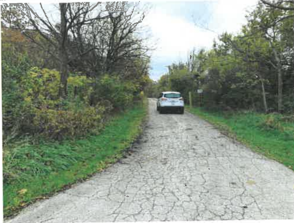
Photo 1: Main Access Road at Minkler Road Facing West
