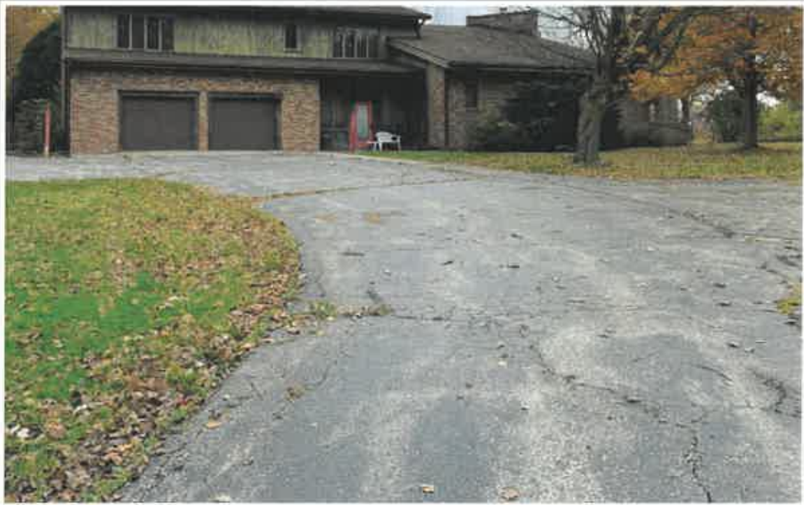
Photo 4: Existing Driveway Facing East
