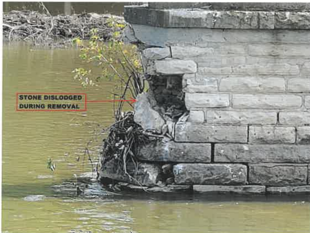
Photo 2_Pier 1-Upstream-Northeast Nose
