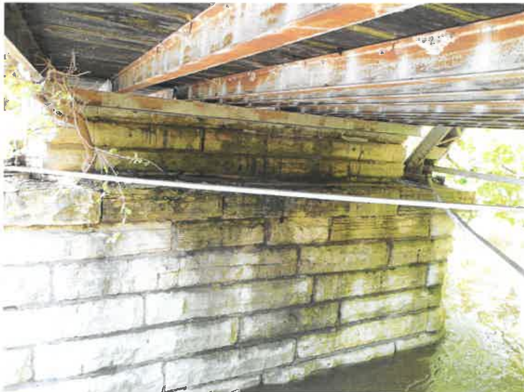
Photo 14_Pier 2-West Face-May 2017
