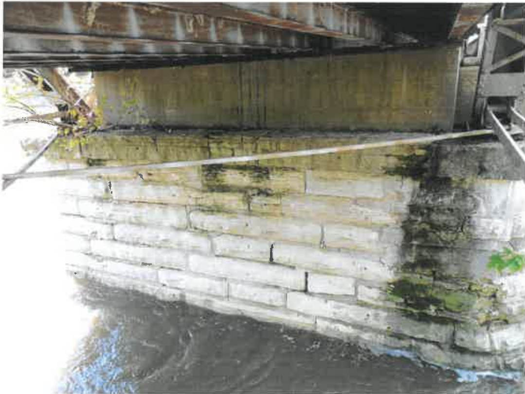
Photo 8_Pier 1-West Face-May 2017
