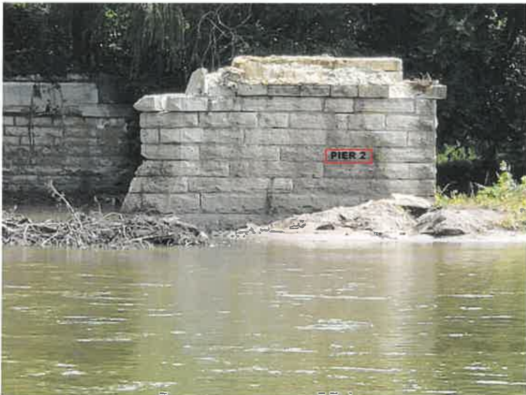
Photo 10_Pier 2-East Elevation
