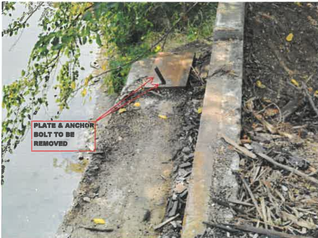
Photo 20_East Abutment-South Bearing Plate-Anchor Bolt
