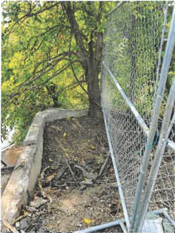
Photo 21_East Abutment-North West Wingwall
