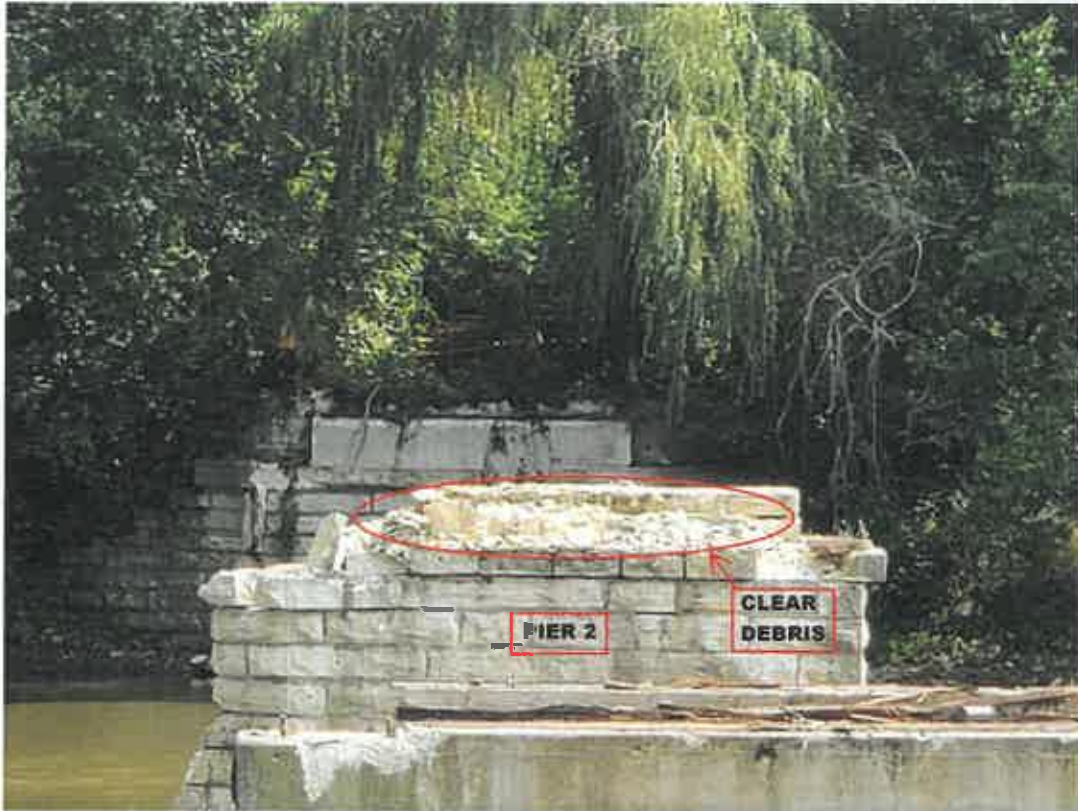
Photo 11_Pier 2-East Face
