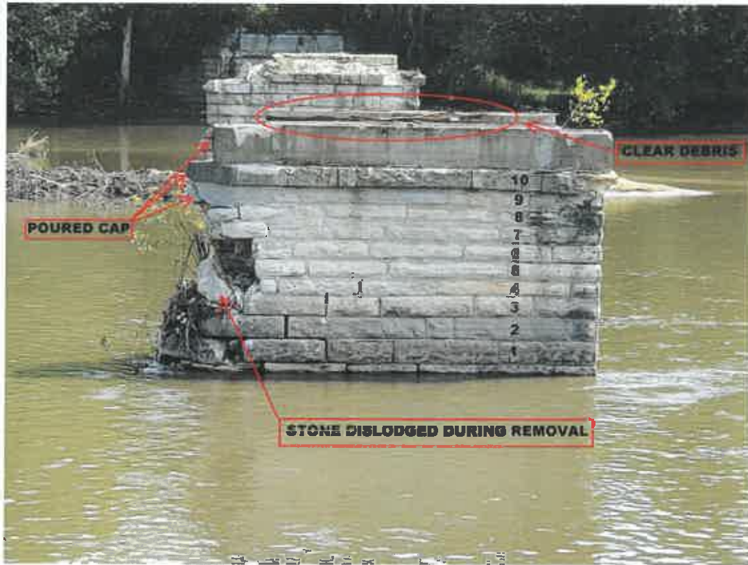
Photo 1_Pier 1-East Elevation
