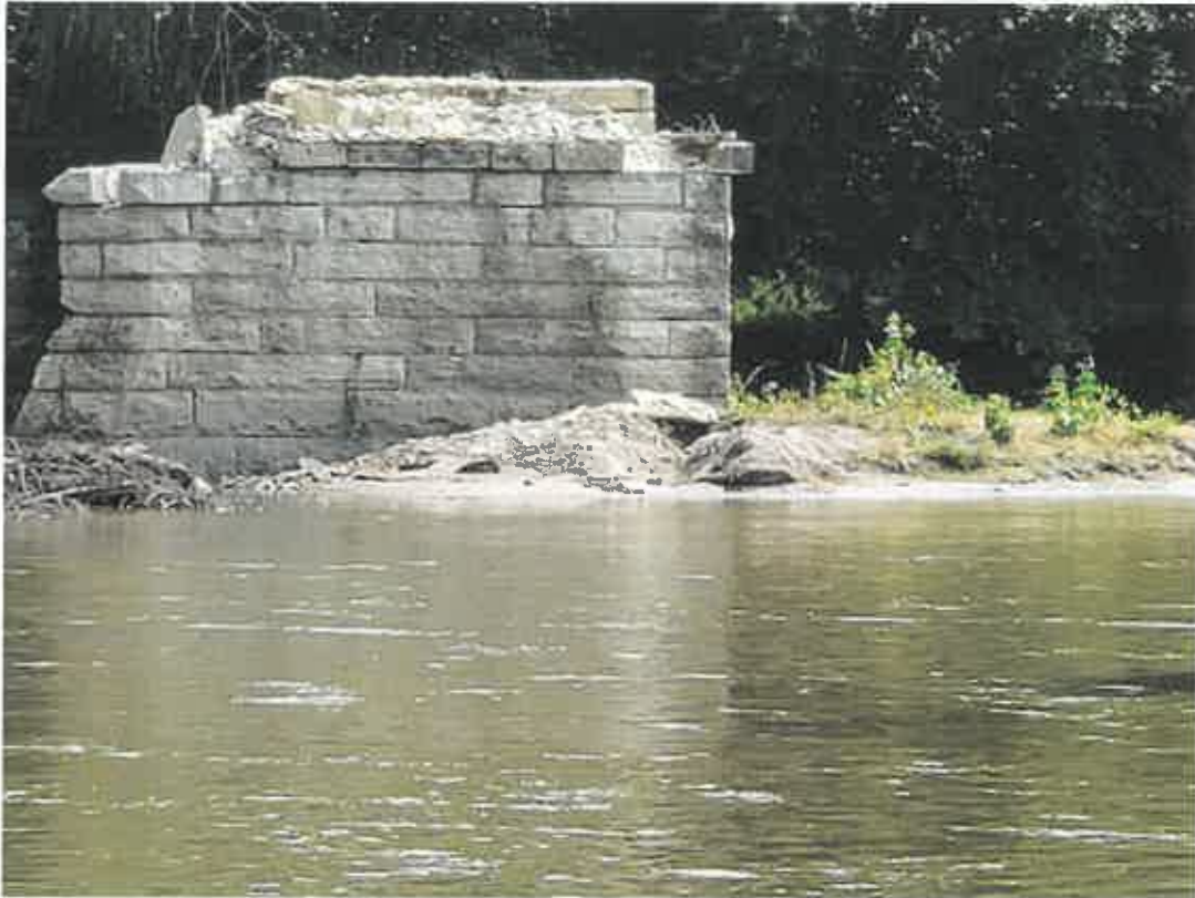
Photo 9_Pier 2-East Elevation
