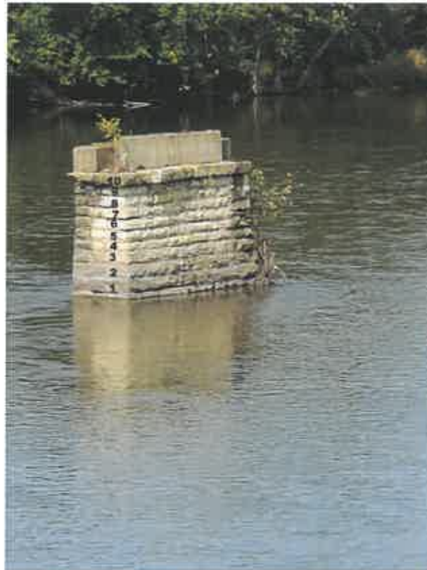
Photo 5_Pier 1-West Face
