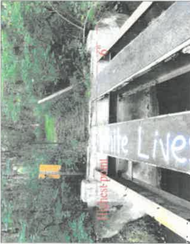
approach built up to match plank height by others
