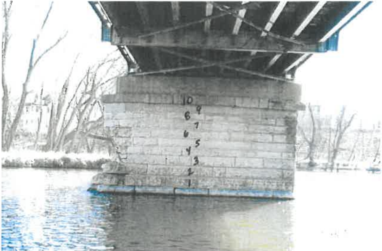
Photo 15_View of Pier 1, Looking East-April 2015
