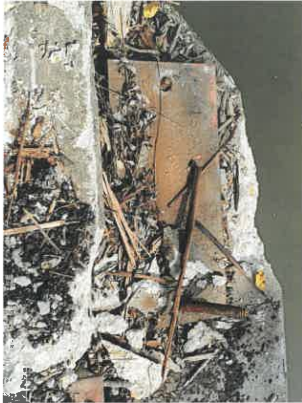
Photo 23_East Abutment-Bearing Seat.
