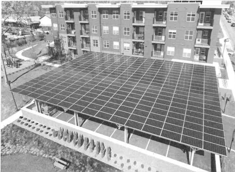
Canopy / Carport Mounted in Indiana
