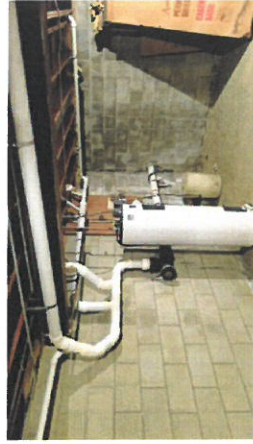
1. View located under proposed new bathrooms with easy plumbing access.
