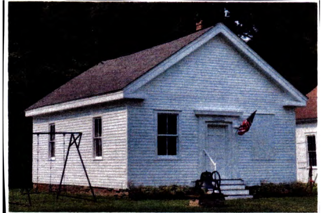
Photo with new staircase
