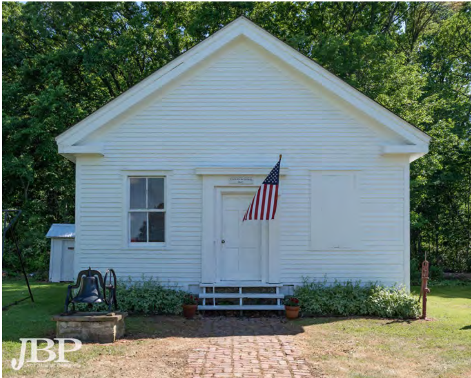
Photo with old staircase
