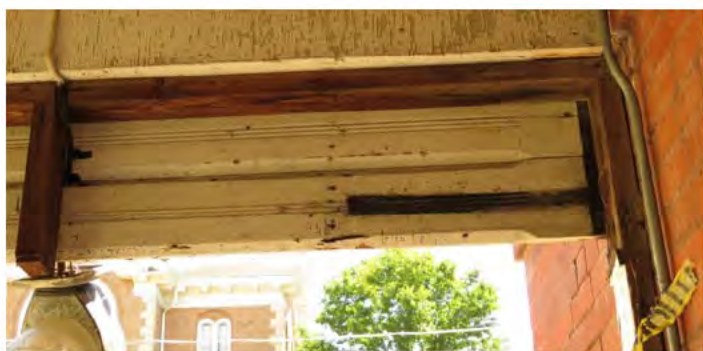
OLD COLUMNS USED AS FASCIA - REINSTALLED AT COLUMNS
