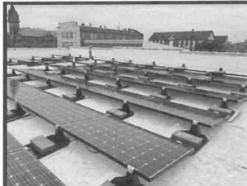
Historic building on Main Street with Solar Panels and no impact on the historic character.
