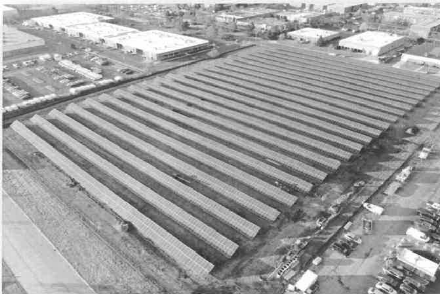
Ground Mounted in Illinois
