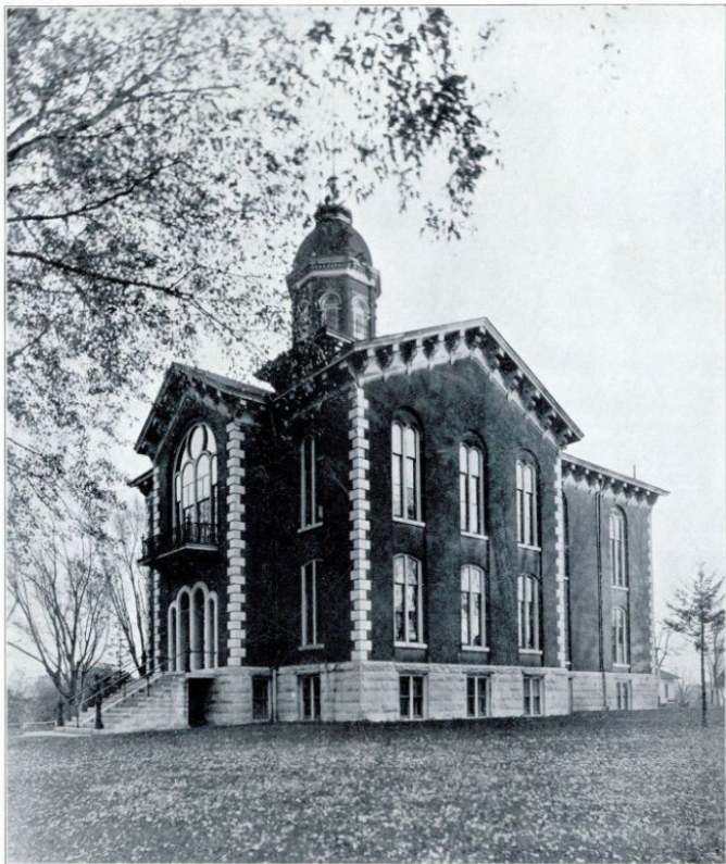
KENDALL COUNTY COURT HOUSE, YORKVILLE, ILLINOIS.
