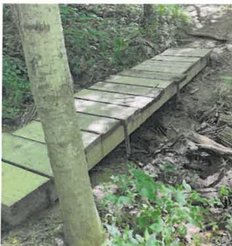
Figure 1: RY Foot Bridge
