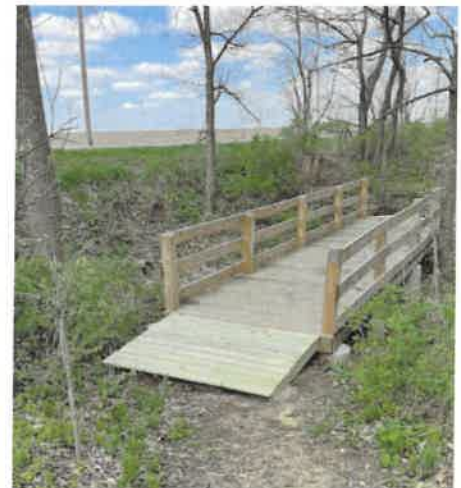
Figure 3: LRC Bridge Ramps
