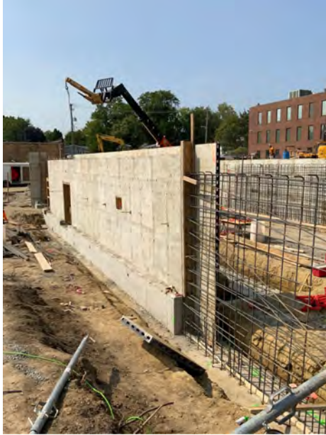
1. East wall with penetrations
