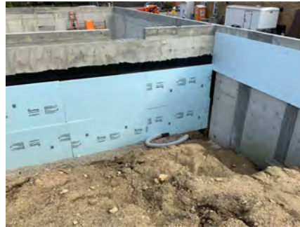
Insulation, DP & Waterproofing
