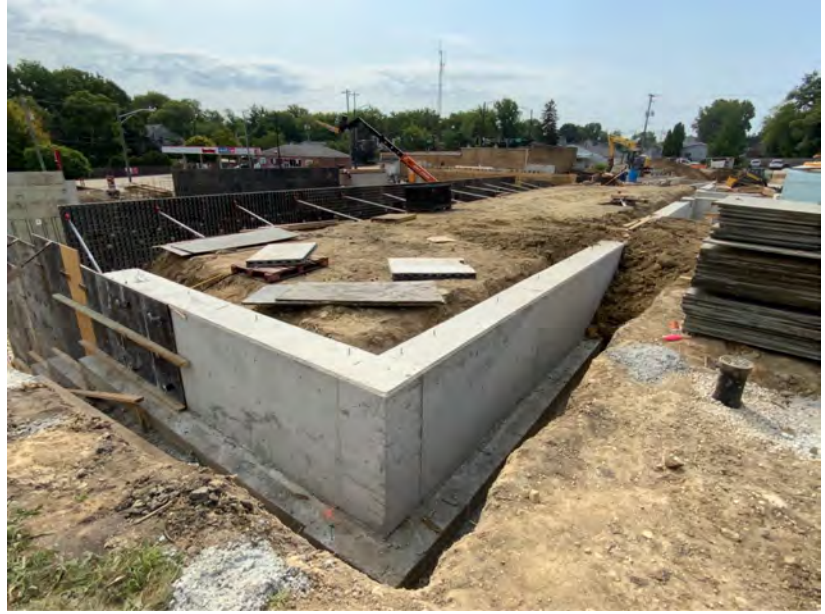
2. Northwest corner foundation wall and footing
