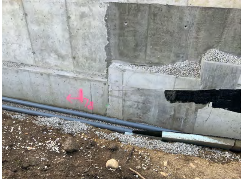
Concrete Ledge at Elevation -10'-0"
