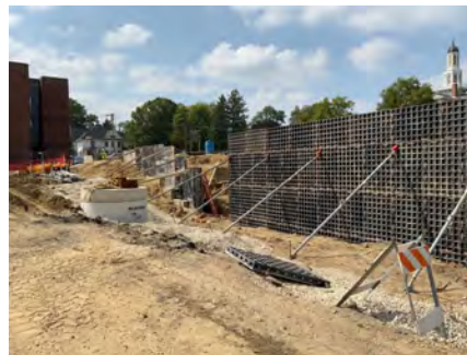
Overall Construction South 1
