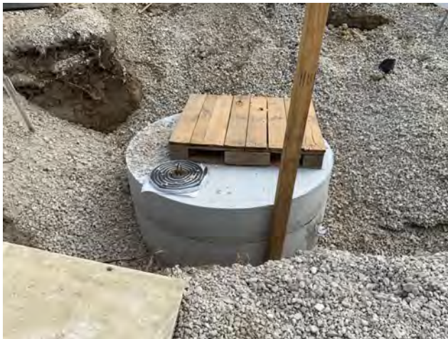
Concrete Storm Structure along South
