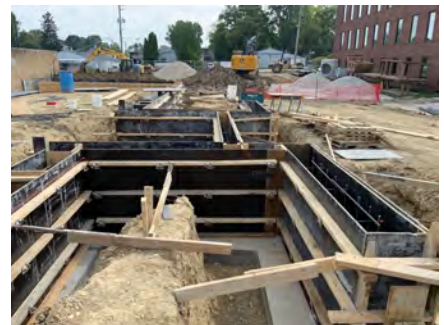
Overall Construction Northeast
