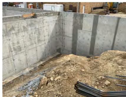
Concrete Foundation Walls
