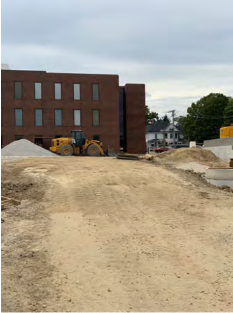
Site Progress at South
