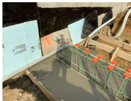
Retaining Wall Intersection
