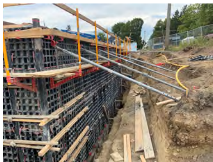
Concrete Frame along North
