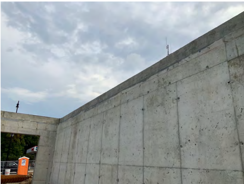
Steel Angle Along Basement Wall Perimeter
