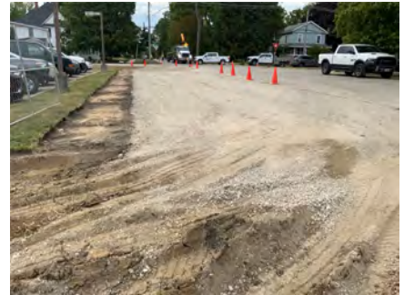
Gravel Base along Ridge St.
