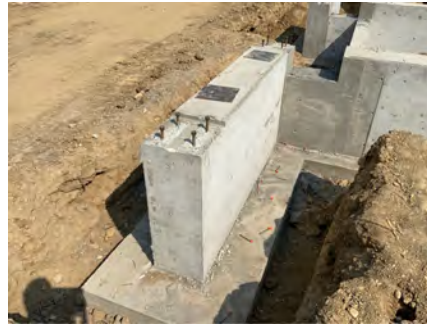
6. Pier at entrance
