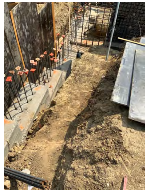
4. North wall stepped footing
