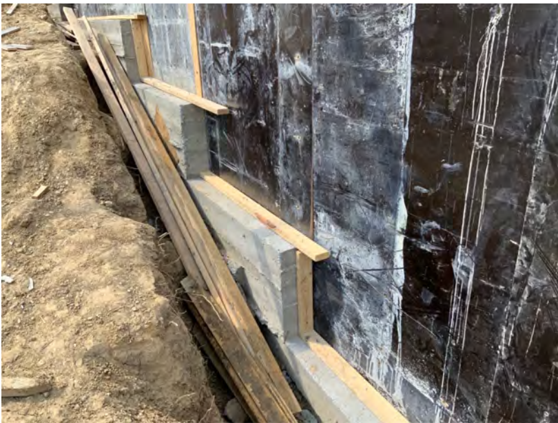
Stepped Foundation along South
