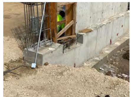
12. Door opening at east wall
