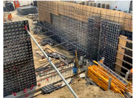
7. Rebar for wall along grid 3
