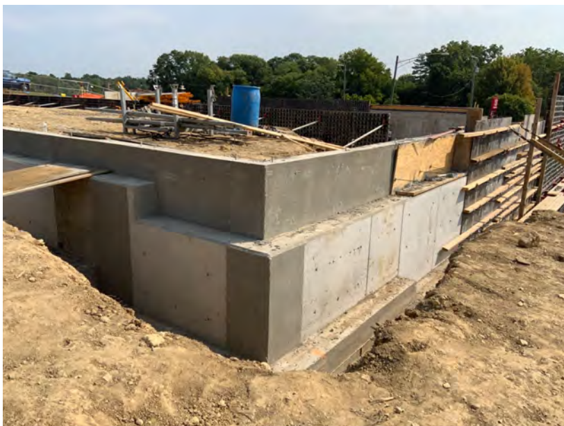
3. Southwest corner foundation wall, ledge, and footing
