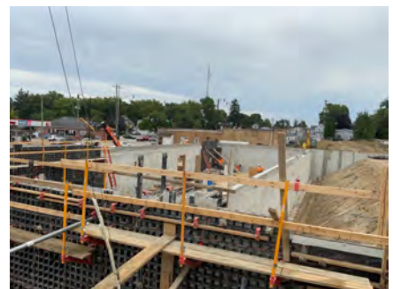
Overall Construction Progress
