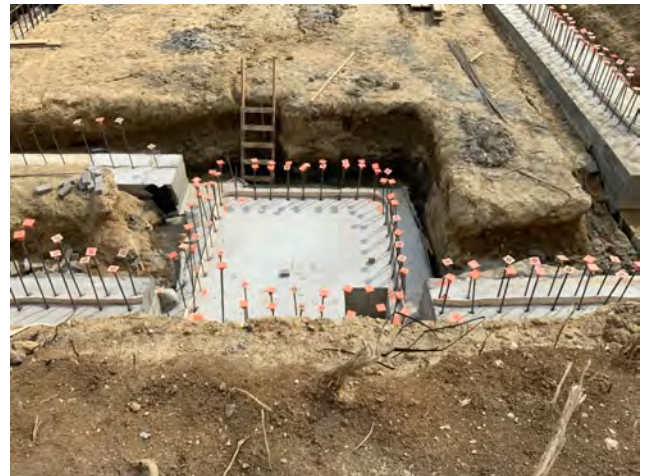
Elevator Pit Slab and Sump Pit
