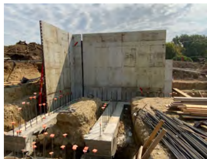
11. Foundation at NE corner
