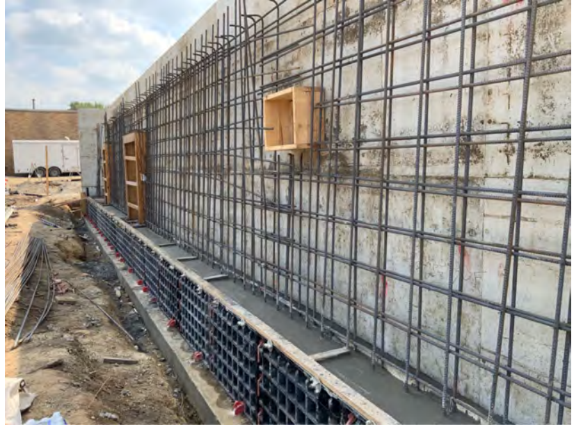
Concrete Foundation Wall, Footing and Ledge along East
