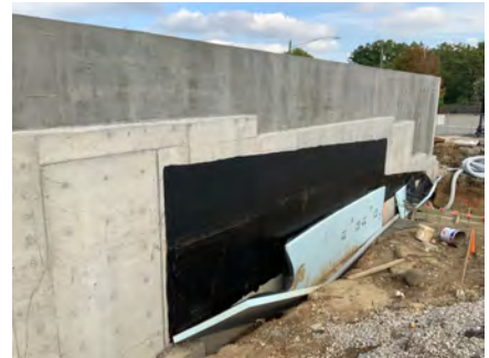
Insulation, DP & Waterproofing
