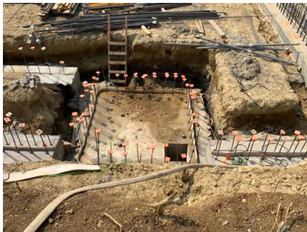
8. Elevator pit slab with sump pit
