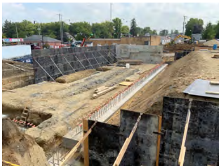
Overall Construction North
