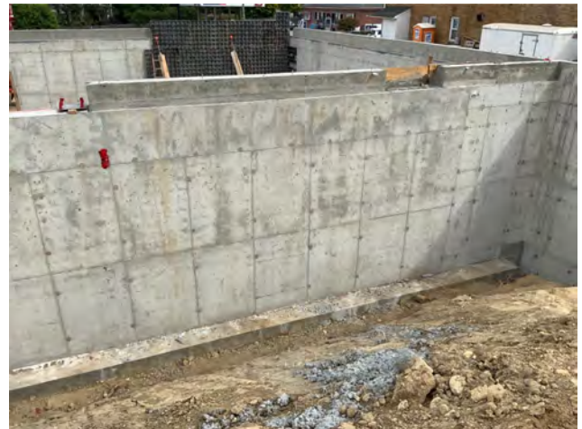
Wall Openings Along Gridline 3
