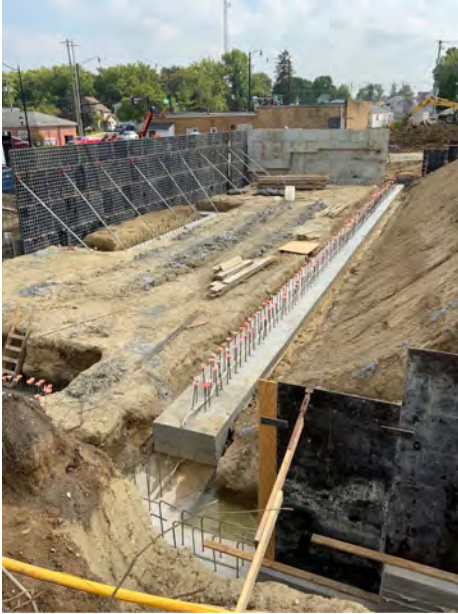
Footing at Gridline 3
