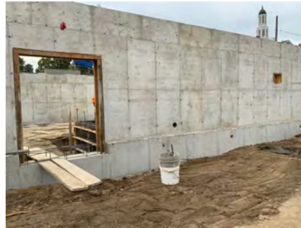
Framed Openings at East
