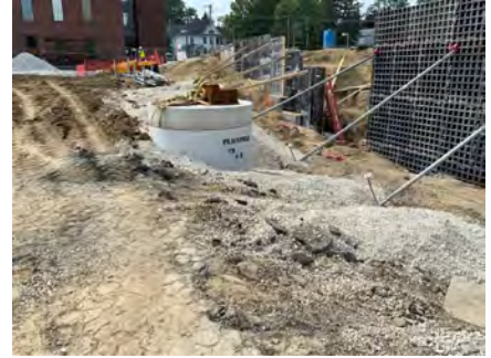
Backfill at Storm Structure
