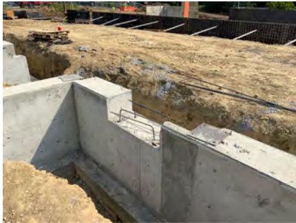
5. Door opening with dowels
