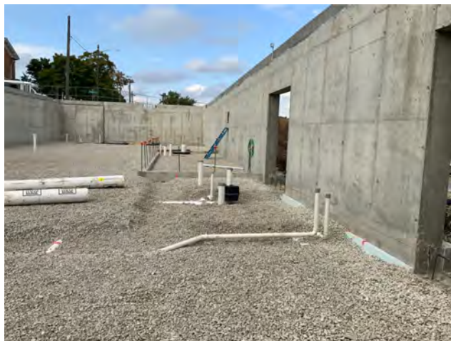
Underground Plumbing Piping & Stone Base
