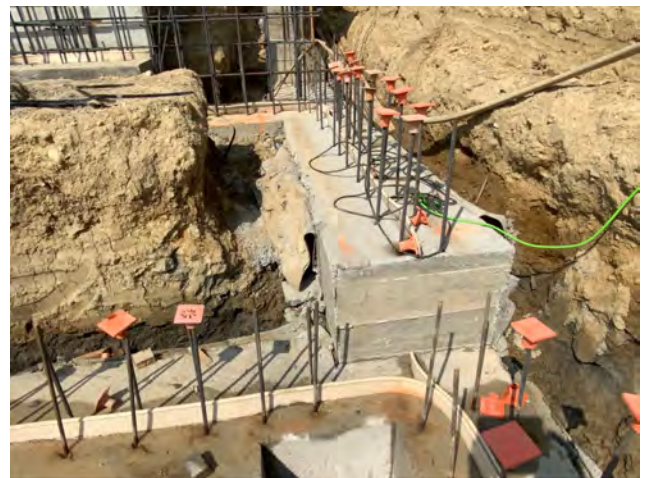
9. Stepped footing connecting to elevator pit
