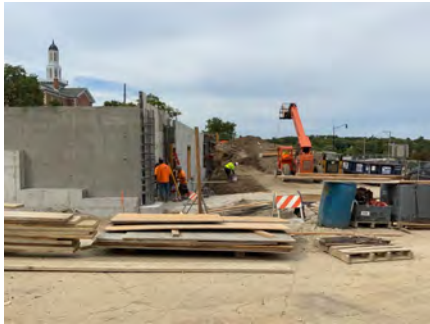
Construction in Progress
