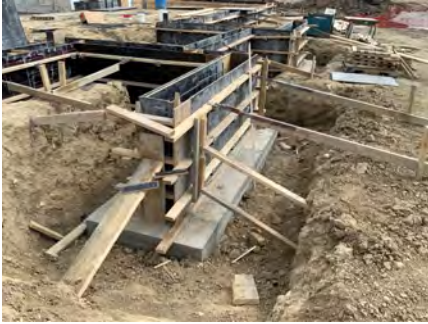
Footing and Wall Prep at West
