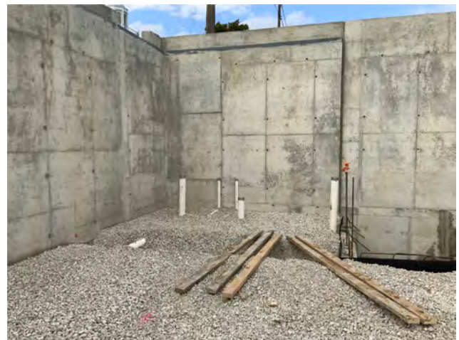
Underground Plumbing Piping Sprinkler Room
