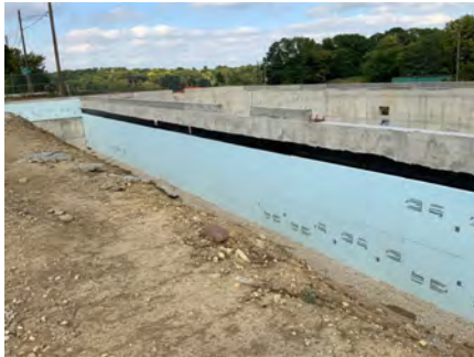
Insulation Along Gridline 3
