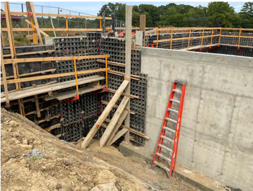
Wall Openings along Gridline 3
