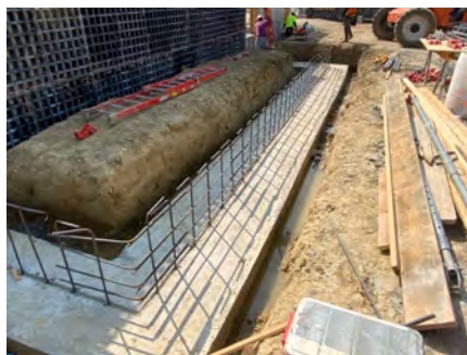
10. Int. CMU wall footing
