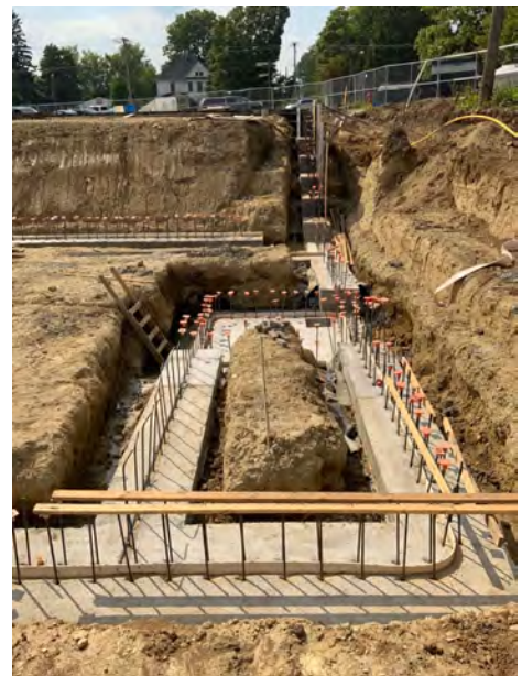
Footings along North for Stair
