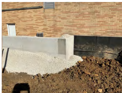
Retaining Wall at Old Fire House
