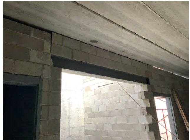
Steel Lintel at Elevator Opening
