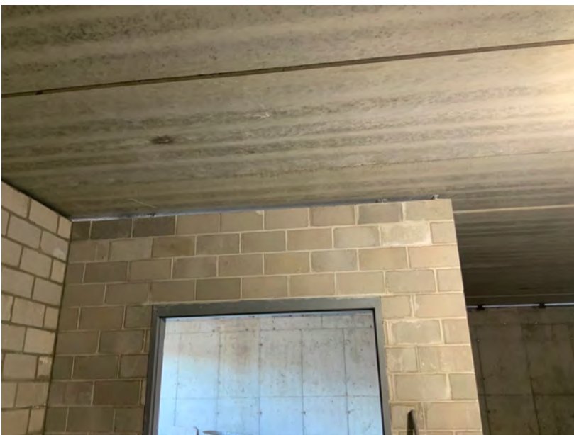
Non Load Bearing CMU Wall in Basement
