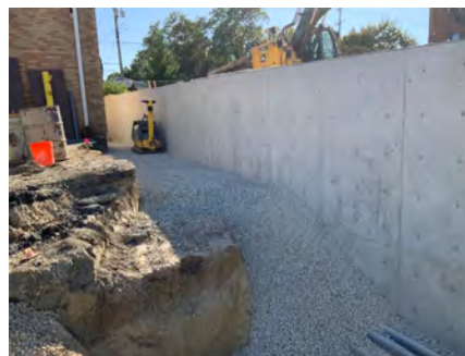
Retaining Wall Progress
