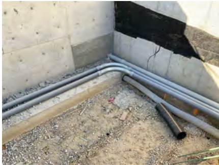
Underground Perimeter Drain
