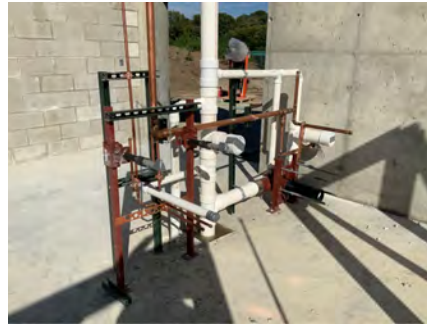
Plumbing Piping Progress
