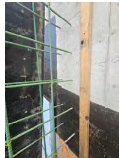
#12 - Retaining Wall Reinforcement
