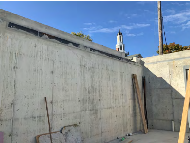
Steel Angle with Holes at Northwest Corner
