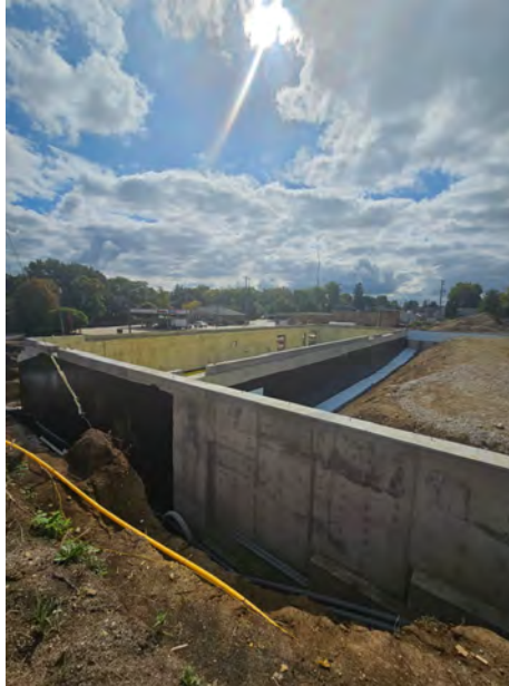
#2 - Wall along grid 3
