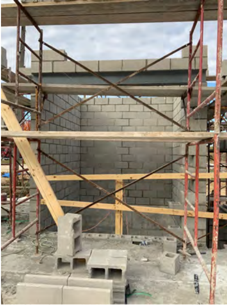
CMU Elev. Shaft and Steel Lintel
