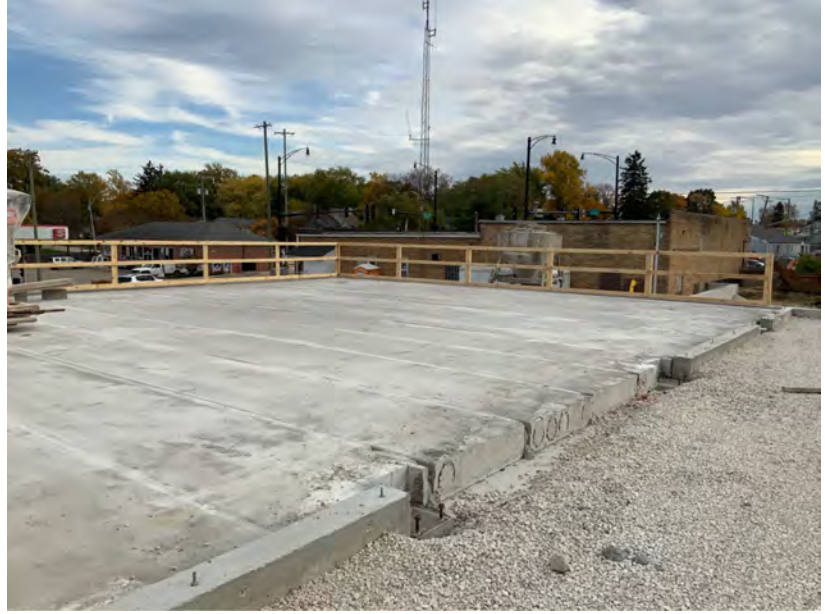
Precast Plank and Aggregate Prep for Slab on Grade
