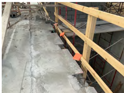
Edge Condition at Stair A
