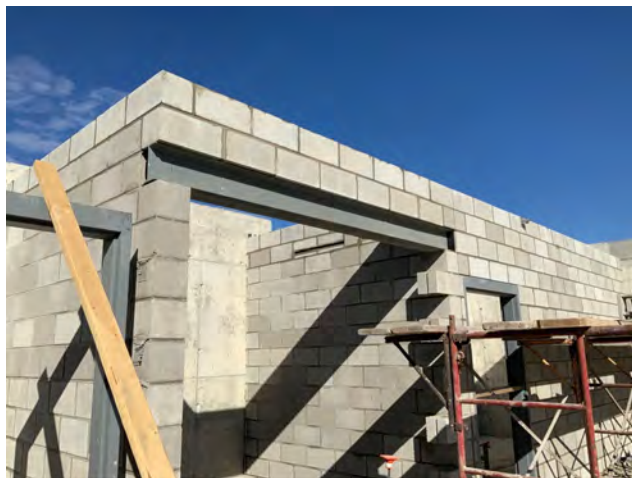
Steel Lintel at Elevator
