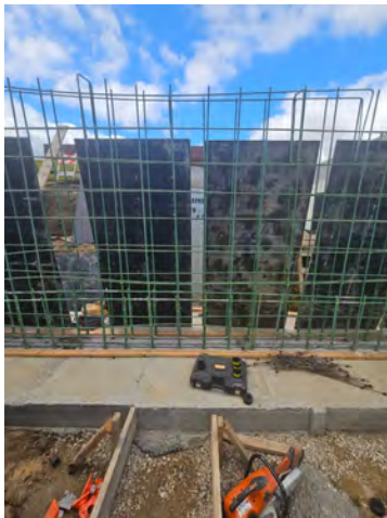
#8 - Retaining Wall Reinforcement
