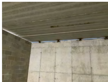
Precast Plank at South
