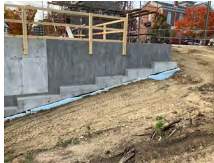
Drainage, Insulation & Backfill
