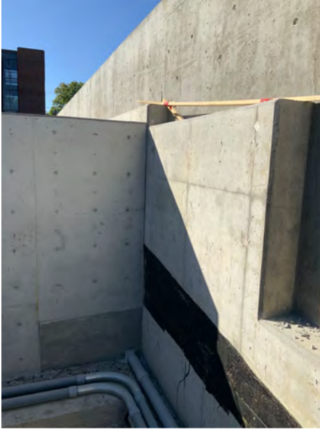
Retaining Wall Intersection End
