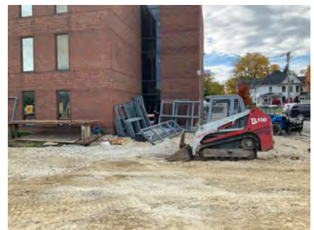
Hollow Metal Frames on Site
