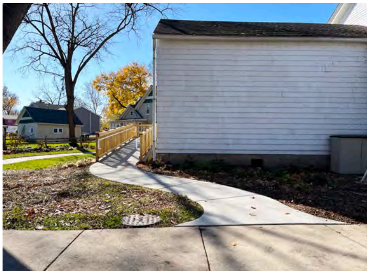
The new accessibility ramp at the Little White School Museum wraps around the 1936 classroom addition to a platform on the south side of the building and a new door. The door panel on the right can be opened to allow large items to be moved in and out of the museum gallery, and a portion of the railing is removable to allow movement of bulky items.
