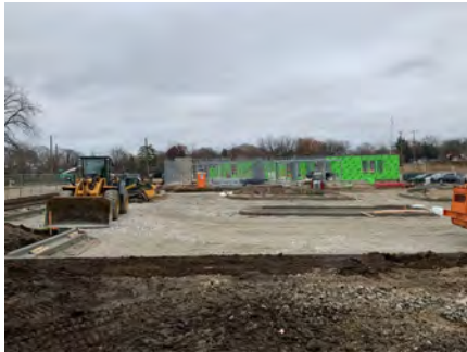
West Parking Lot Progress
