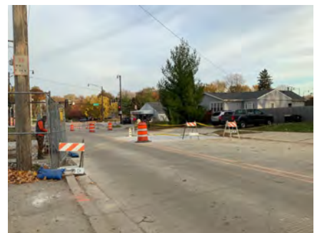
Water Main Connection Work
