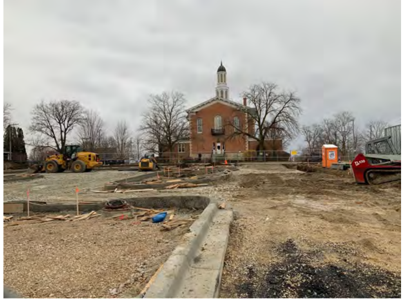
Curbs and Gutters along West Drive
