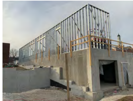
Overall Progress of Framing
