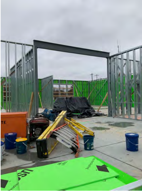
Steel Beam and Columns along 3
