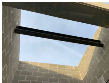
Steel Beam for Hoistway
