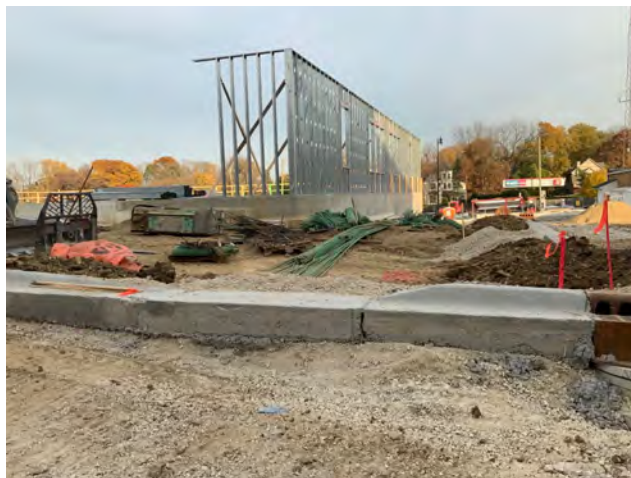
Curb Cut at Accessible Path
