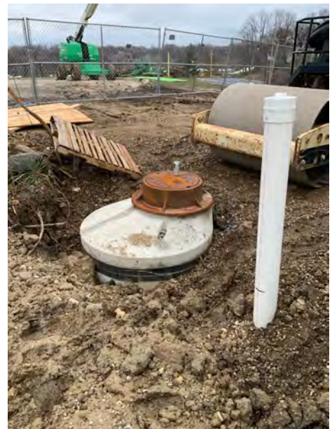
Plumbing Pipe Stub Up on North
