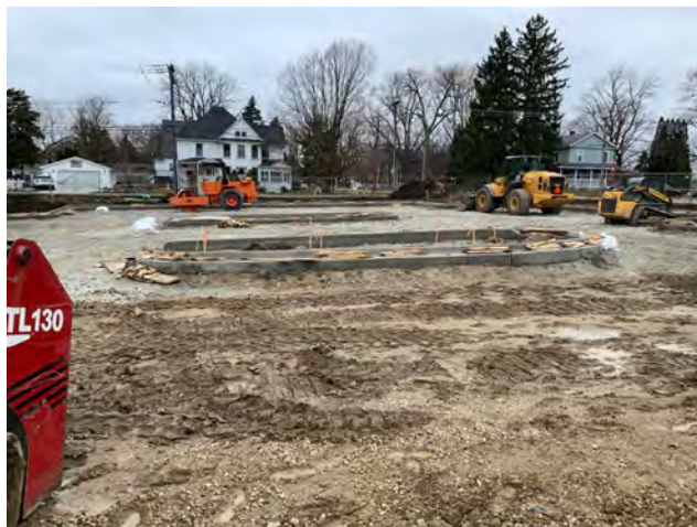
Curb Grading at West Lot Island
