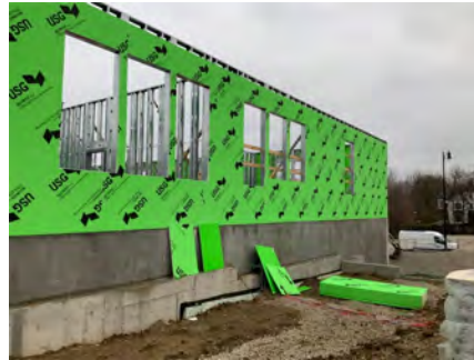
Sheathing & Conduits on South
