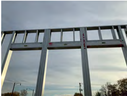
Metal Stud Window Head
