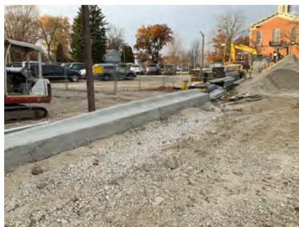
Curb Gutter Extent at West Lot
