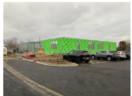
Overall Building Progress
