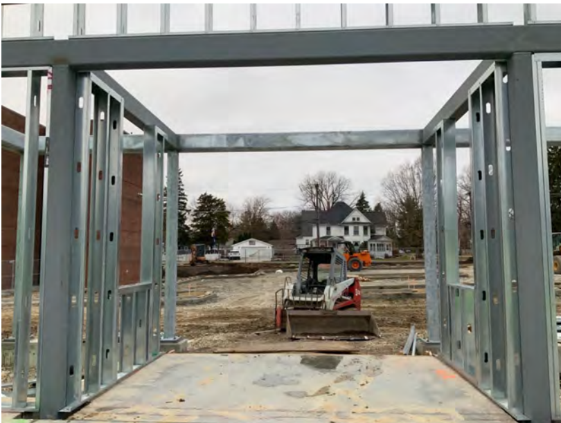
Steel Beams and Columns at Entry
