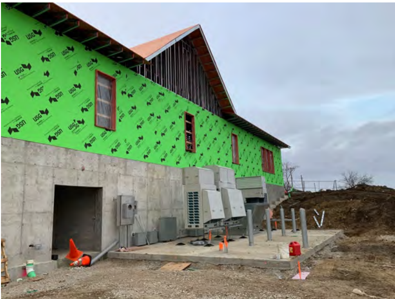
Equipment Pad and Progress on East
