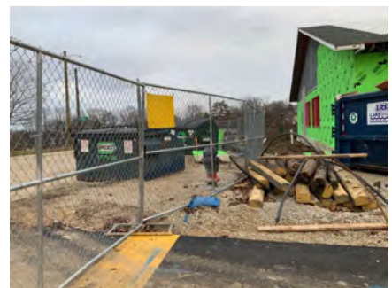
Fire Hydrant on West
