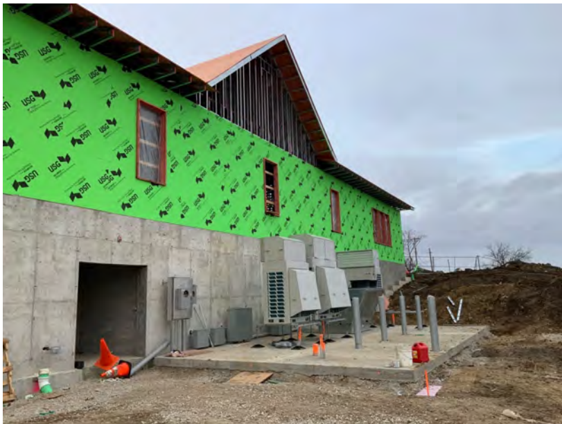
Equipment Pad and Progress on East
