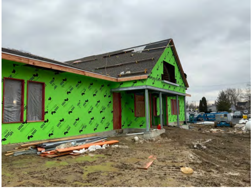
Roof Shingle Progress
