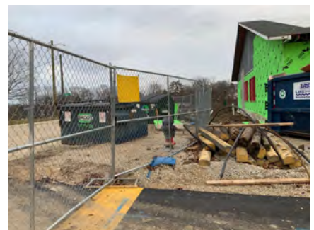
Fire Hydrant on West
