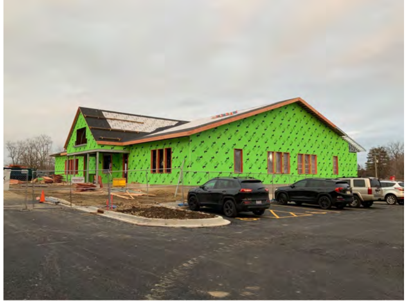
Roof Sheathing and Underlayment Progress on South
