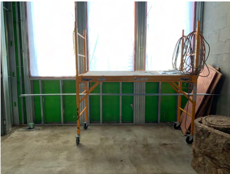
Piping Stub Up in Voter Office 105
