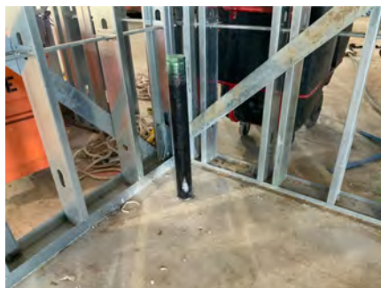
Stub Up in Staging/ Work Area
