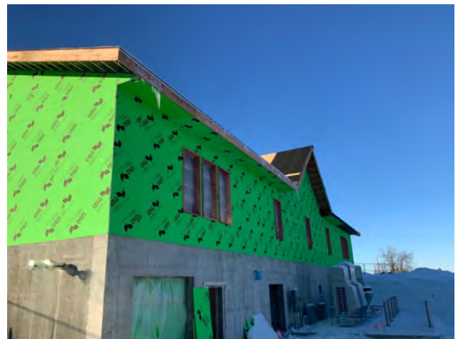
Soffits and East Side
