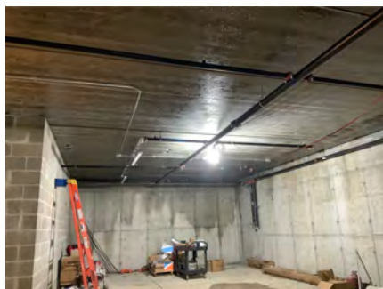
Lighting Progress in Basement
