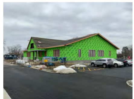
Overall Progress View
