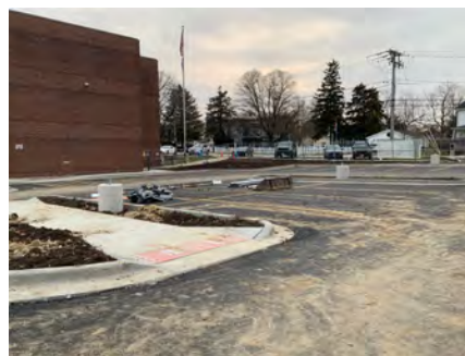
Site Lighting on West
