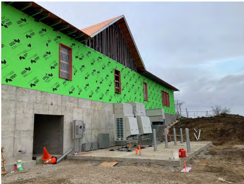
Equipment Pad and Progress on East
