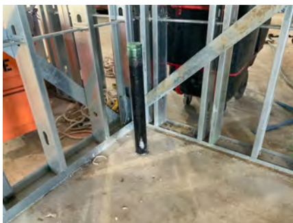
Stub Up in Staging/ Work Area
