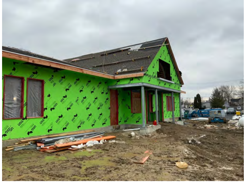
Roof Shingle Progress
