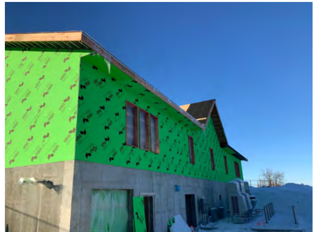
Soffits and East Side
