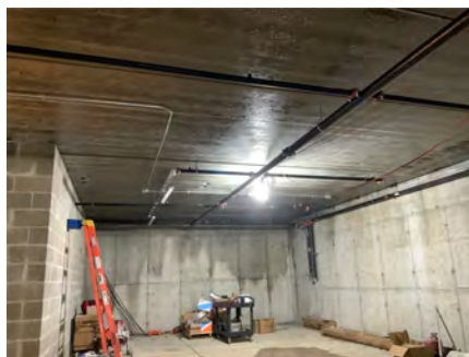
Lighting Progress in Basement
