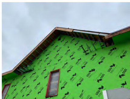
Roof Return Framing
