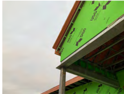
Fascia at Entry Gable
