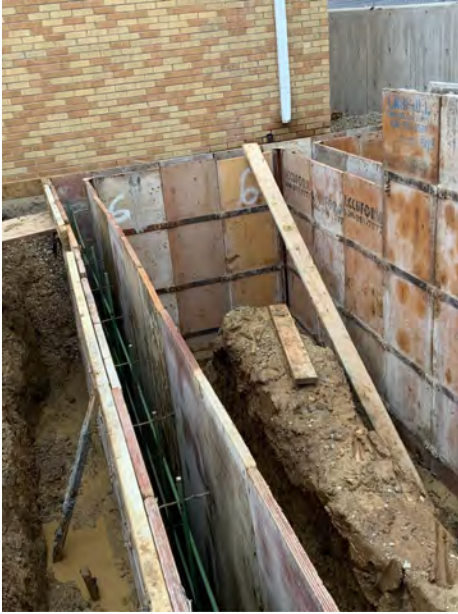
Ramp Foundation Preparation
