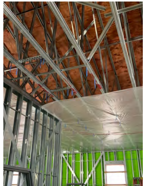
Plastic Sheeting Installation
