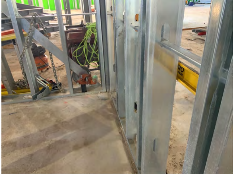
Piping Stub Up in Toilet 6
