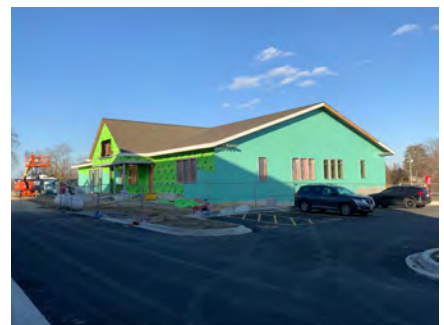
Overall Progress View
