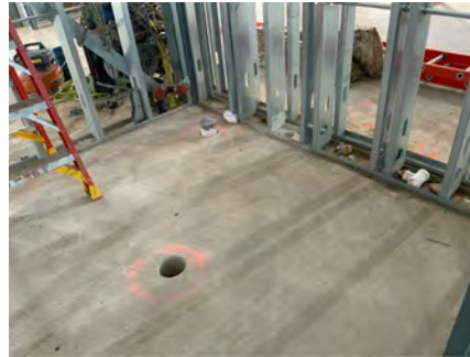
Cores for Plumbing Rough-in
