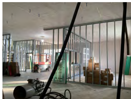
Wall Framing at Library
