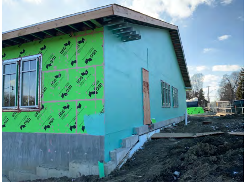
AVM Barrier and Taping/Sealing Progress
