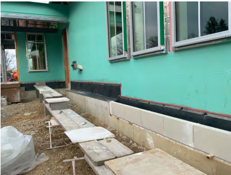
Stone, Flashing, Termination, and Sealant Installation
