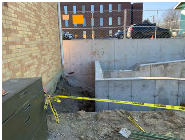
South Ramp Foundation Wall
