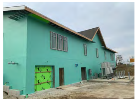
Exterior View from Southeast
