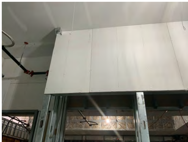
Coiling Grille Location at Recorder Reception
