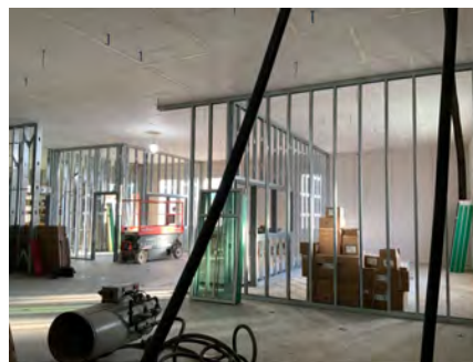
Wall Framing at Library
