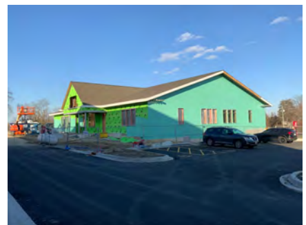
Overall Progress View
