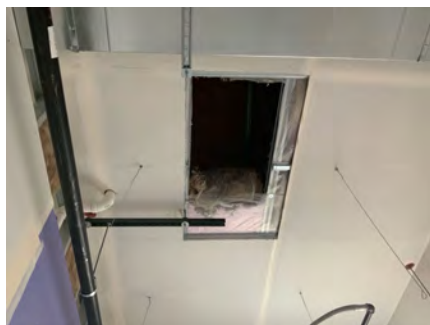
Attic Cap Ceiling Access
