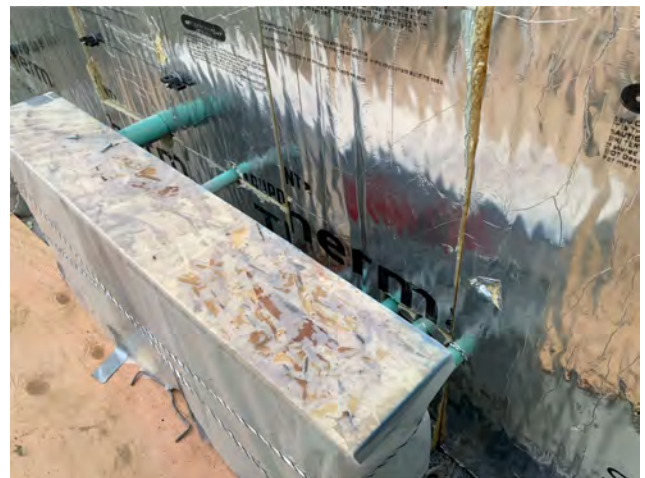
Pipe Penetrations through Polyiso Insulation
