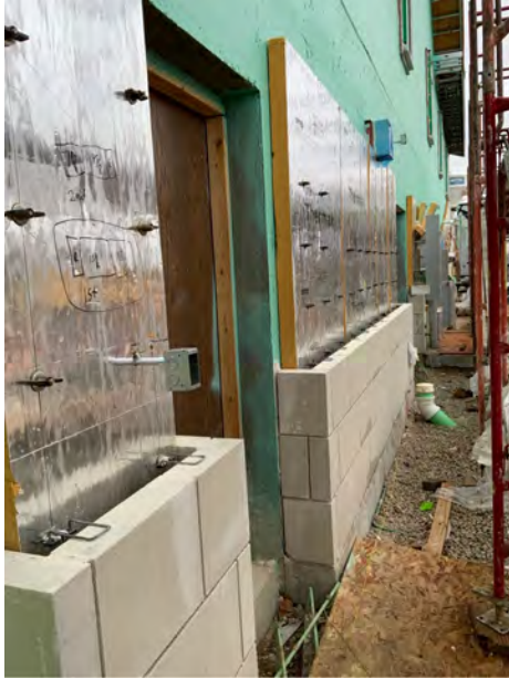
Cast Stone Installation on East
