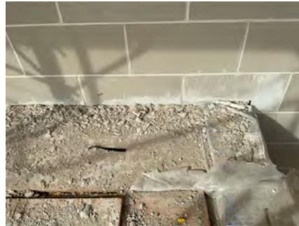
Weeps at Top of Ramp Landing
