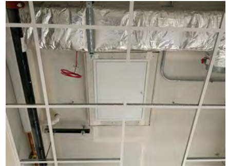
Attic Ceiling Access Panel
