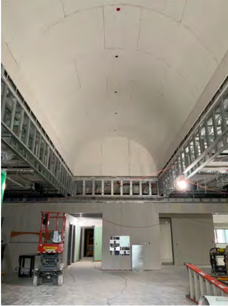
Gypsum Board in Barrel Vault
