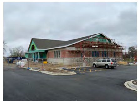
Overall Progress from Southwest
