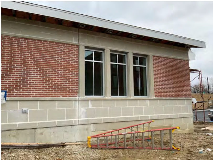
Cast Stone and Brick Veneer on the South West
