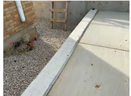
Chamfer Edges along Ramp
