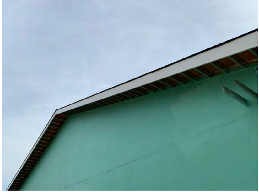
Aluminum Fascia Replacement on North
