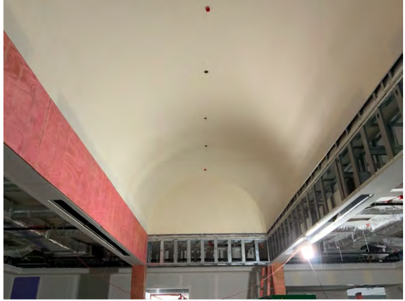
Barrel Vault Ceiling Progress in Lobby
