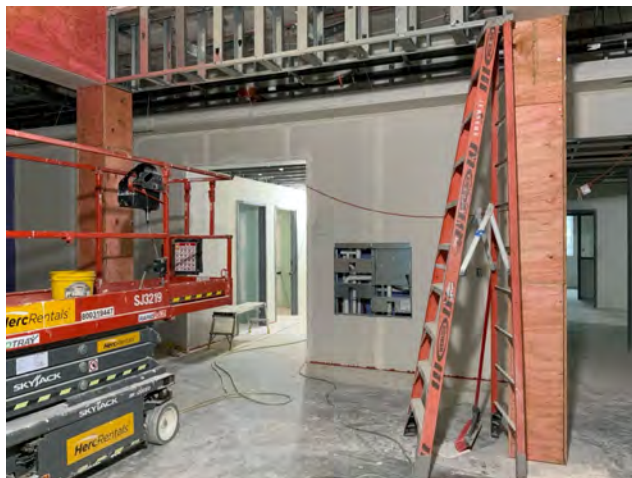
Plywood Columns at End of Barrel Vault
