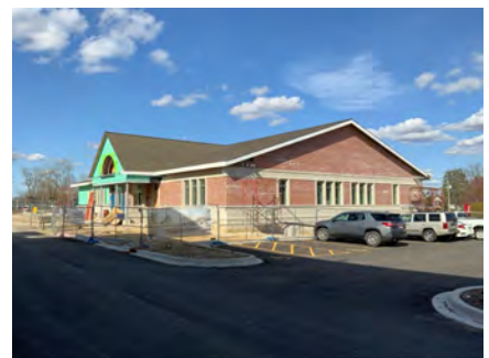
Overall Progress View
