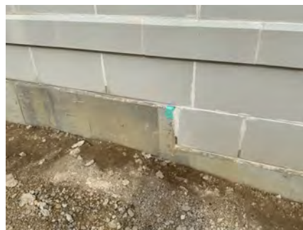
AVM Barrier on Exposed Conc.
