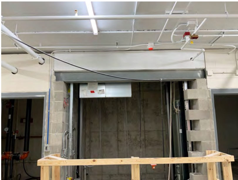
Steel Lintel at Elevator Shaft in Basement
