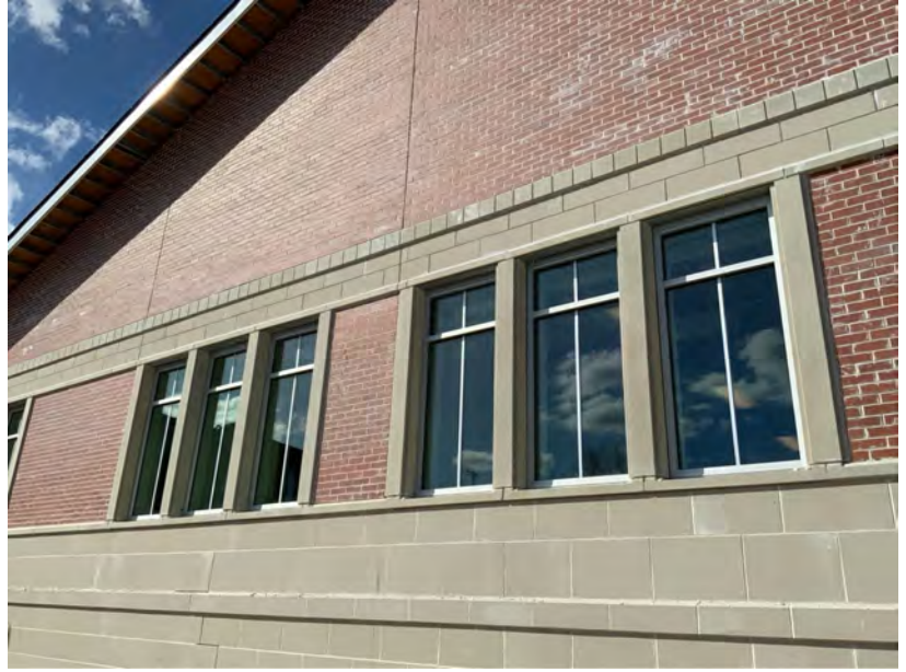
South Facade - Cast Stone and Brick Veneer
