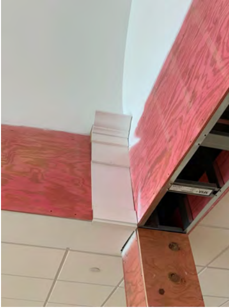
Decorative Trim Mock-up
