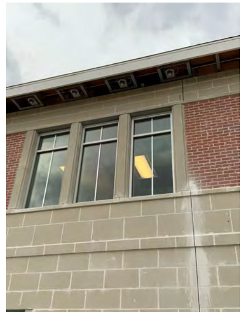
Control Joint on East
