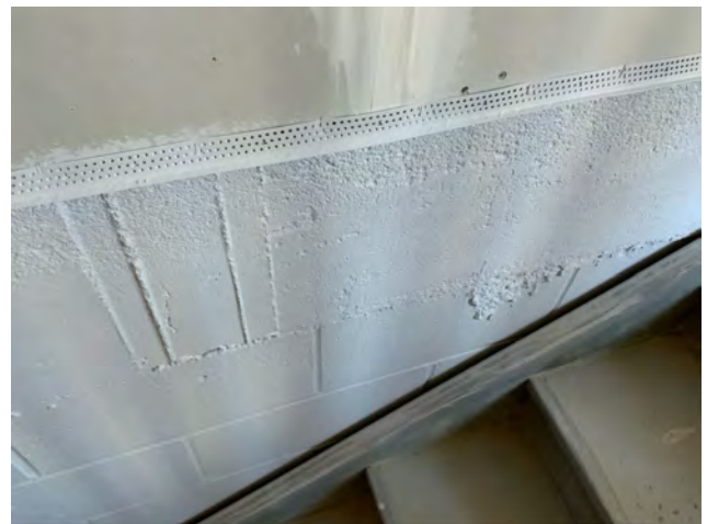
Rough CMU in Stair 1A
