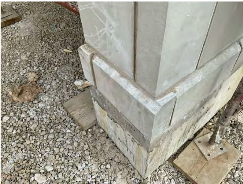
Chamfer Corners of Column Pedestal
