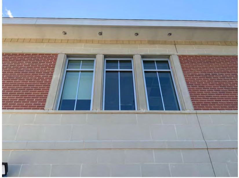
Soffit Cut around Light
