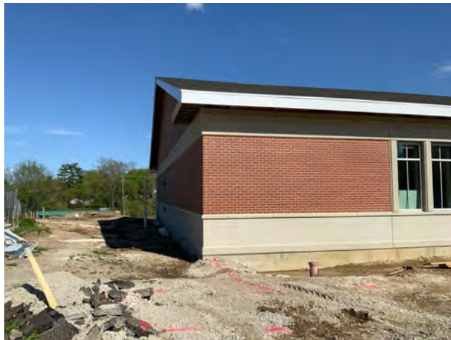
Fascia and Trim on Northwest
