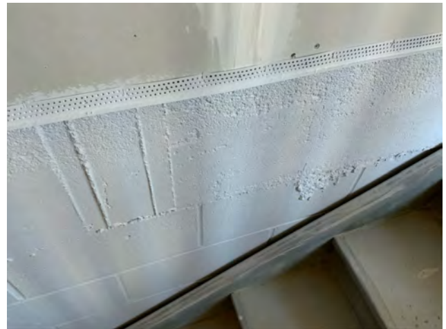
Rough CMU in Stair 1A
