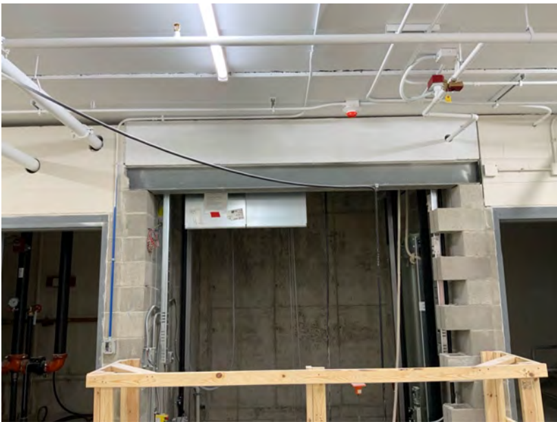
Steel Lintel at Elevator Shaft in Basement
