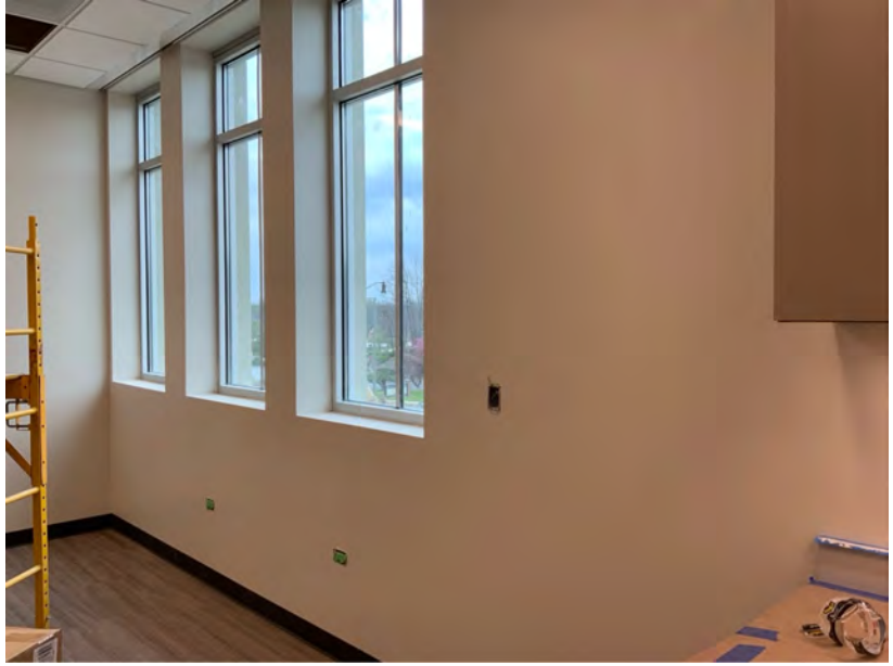
Window Shade Control in Break Room
