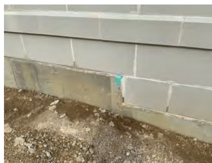
AVM Barrier on Exposed Conc.
