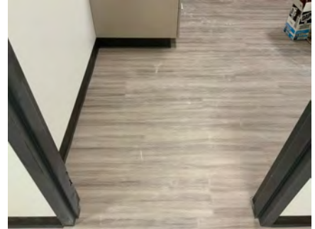
Door Clearance in Work Room
