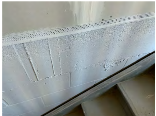
Rough CMU in Stair 1A
