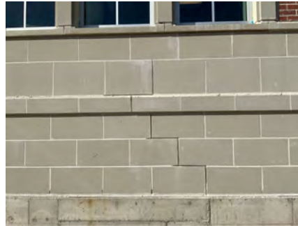
Mortar Joints on South Facade
