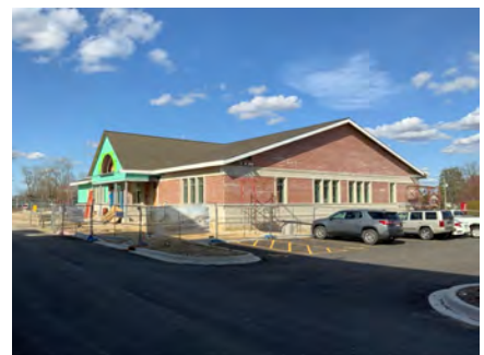
Overall Progress View
