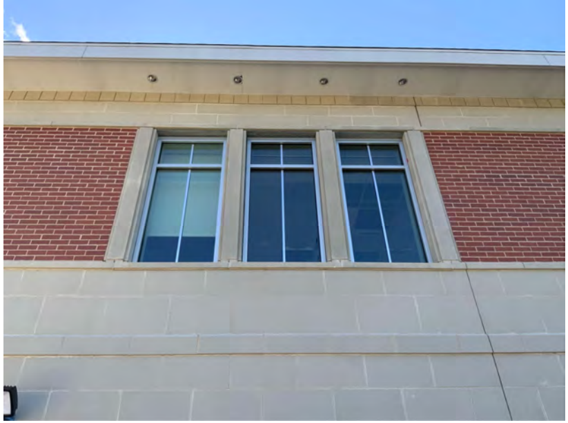
Soffit Cut around Light
