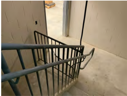
Guardrail Return in Stair
