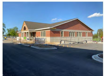
Overall Progress View
