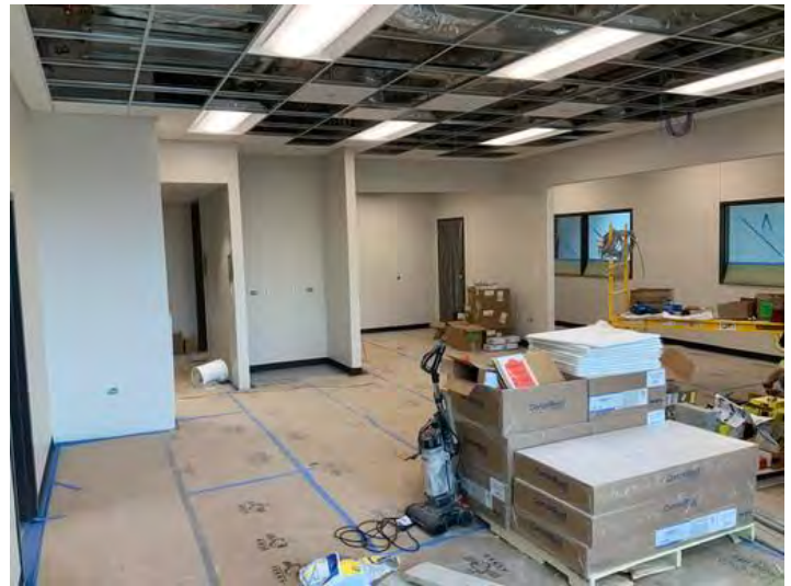
IMG_1787 Taken on Apr 29, 2024, 1:38 PM CDT Added on Apr 30, 2024, 4:48 PM CDT Added by Ken Gleason
