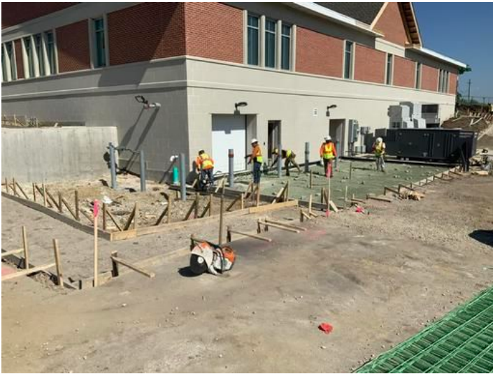
Drive Pad and Sidewalk Southeast Corner
