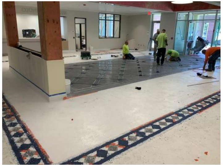
Lobby Terrazzo Flooring
