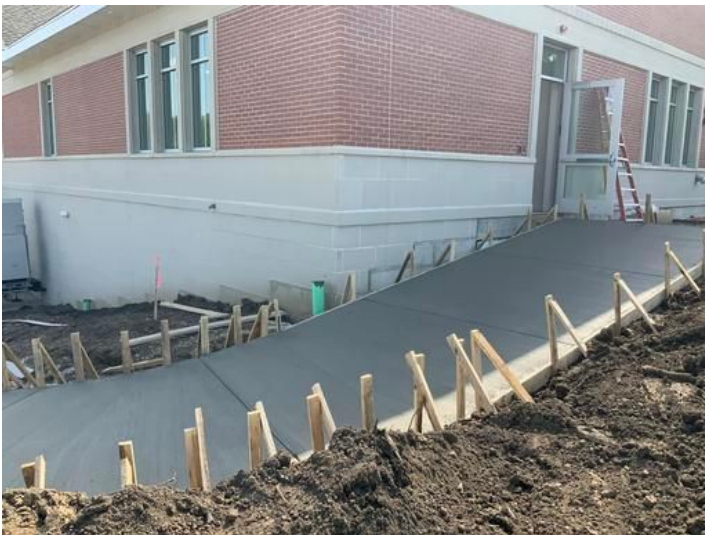
Drive Pad NE Corner
