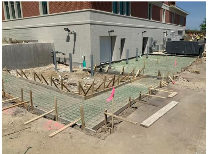
Drive Pad and Sidewalk SE Corner
