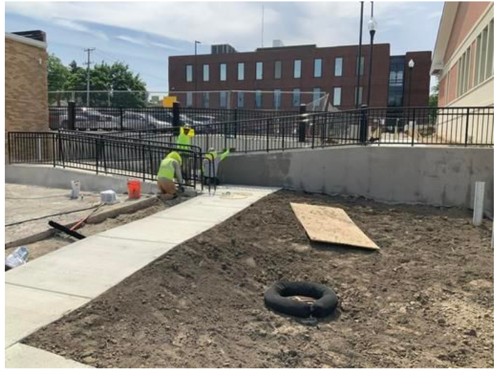
Rubbed finish install at ADA ramp Taken on May 31, 2024, 3:26 PM CDT Added on May 31, 2024, 3:41 PM CDT Added by Ken Gleason
