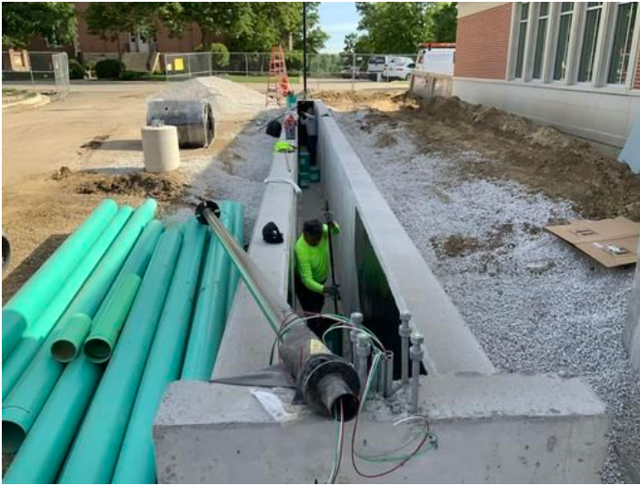
Planter box with waterproofing work Taken on May 31, 2024, 8:25 AM CDT Added on May 31, 2024, 3:41 PM CDT Added by Ken Gleason
