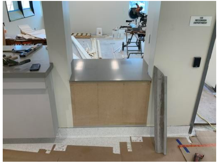
Counter top install at lobby Taken on May 31, 2024, 3:17 PM CDT Added on May 31, 2024, 3:41 PM CDT Added by Ken Gleason
