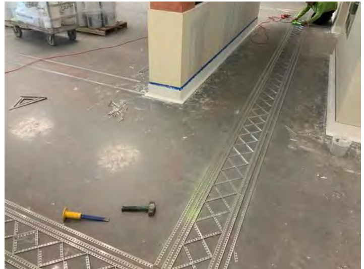
Lobby Terrazzo Tracks Taken on May 10, 2024, 1:03 PM CDT Added on May 10, 2024, 1:18 PM CDT Added by Ken Gleason
