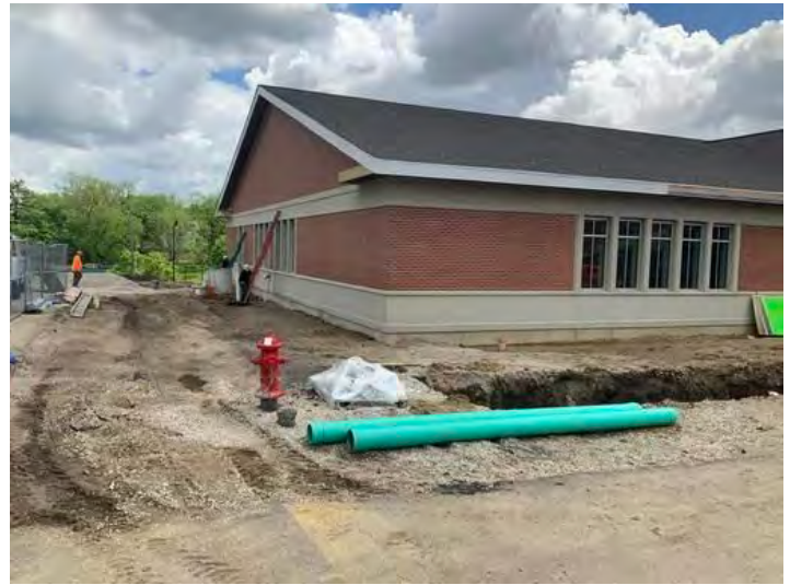
Expansion Joint Filling Taken on May 10, 2024, 12:58 PM CDT Added on May 10, 2024, 1:17 PM CDT Added by Ken Gleason
