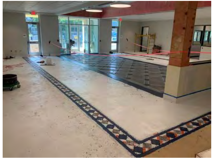
Lobby Terrazzo Flooring
