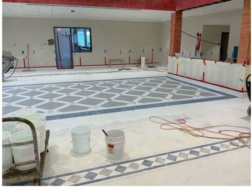
Resinous Terrazzo Floor Progress
