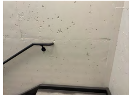
Concrete Wall Finish in Stair
