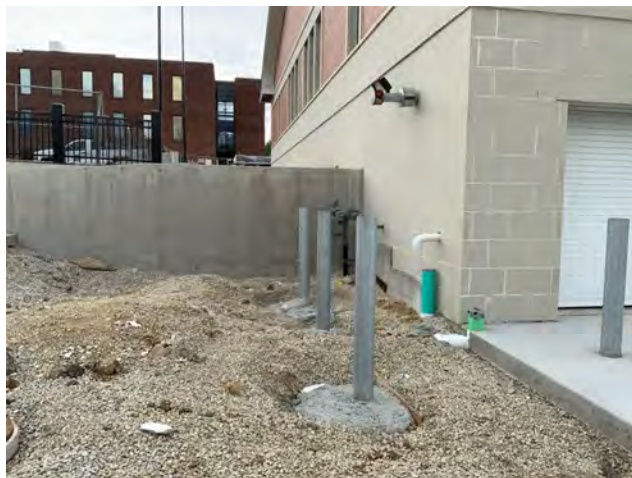
Bollards on Southeast Corner
