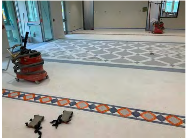
Lobby Terrazzo Flooring
