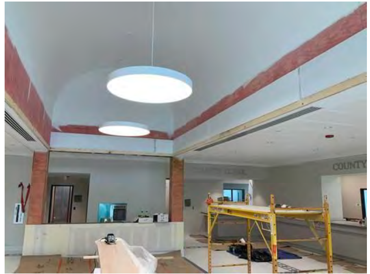
Flatstock trim being installed at lobby Taken on May 31, 2024, 3:16 PM CDT Added on May 31, 2024, 3:41 PM CDT Added by Ken Gleason
