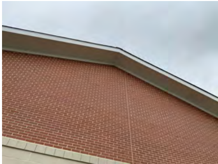
Soffit Panels at Gable
