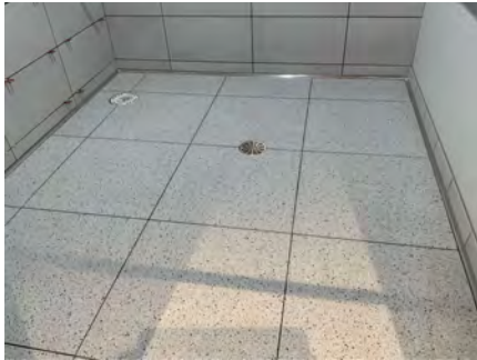
Ceramic Tiling in Toilet Rooms
