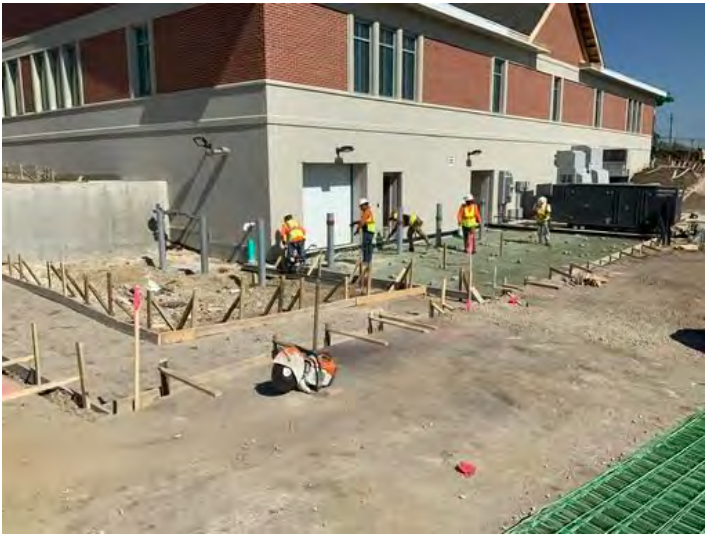
Drive Pad and Sidewalk Southeast Corner
