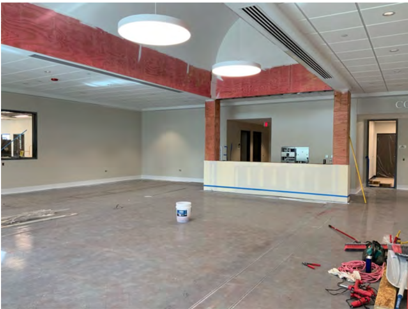
Resinous Terrazzo Progress in Lobby
