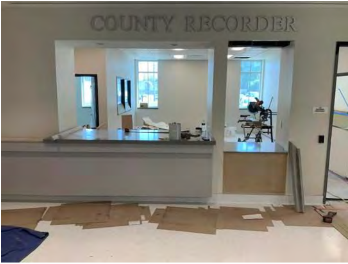
Countertop install in lobby Taken on May 31, 2024, 3:17 PM CDT Added on May 31, 2024, 3:41 PM CDT Added by Ken Gleason
