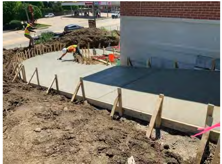
Drive Ramp NE Corner
