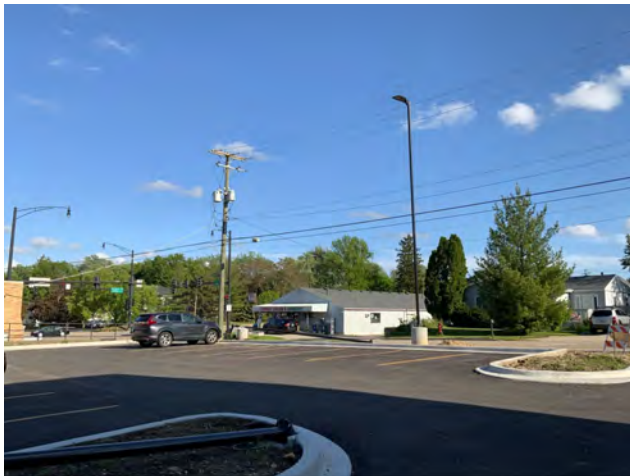
Light Poles near Overhead Power Lines
