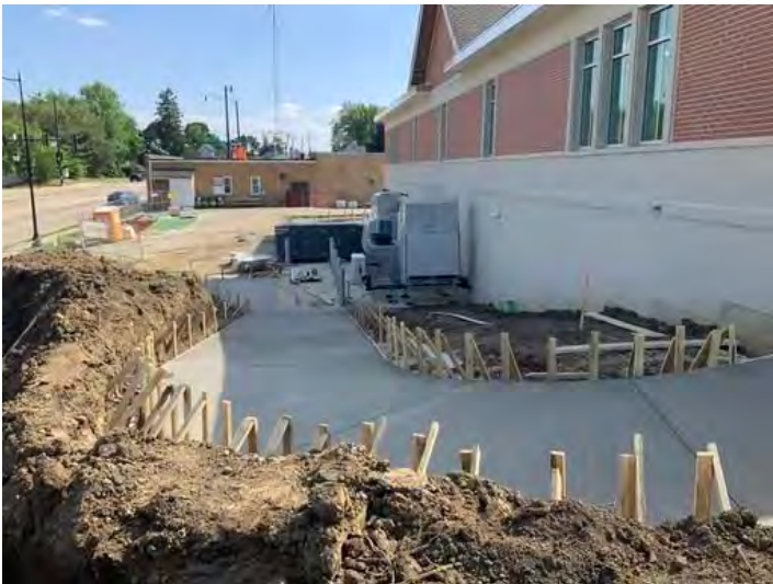
Drive Ramp NE Corner
