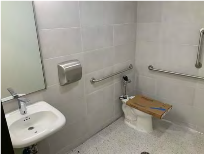
First Floor Bathrooms
