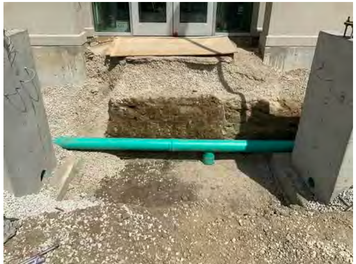
Roof drain tile being installed Taken on May 31, 2024, 3:13 PM CDT Added on May 31, 2024, 3:41 PM CDT Added by Ken Gleason
