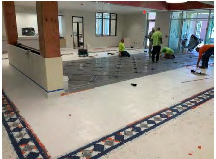
Lobby Terrazzo Flooring
