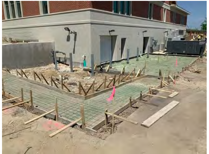
Drive Pad and Sidewalk SE Corner
