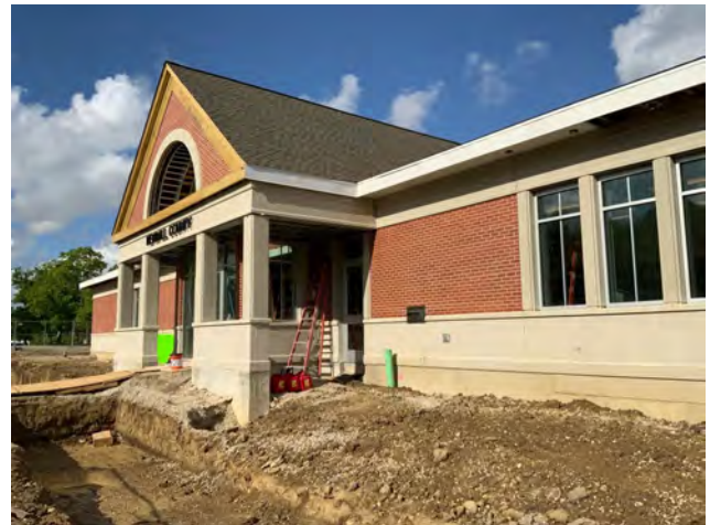
Wood Trim and Kendall County Sign at Gable
