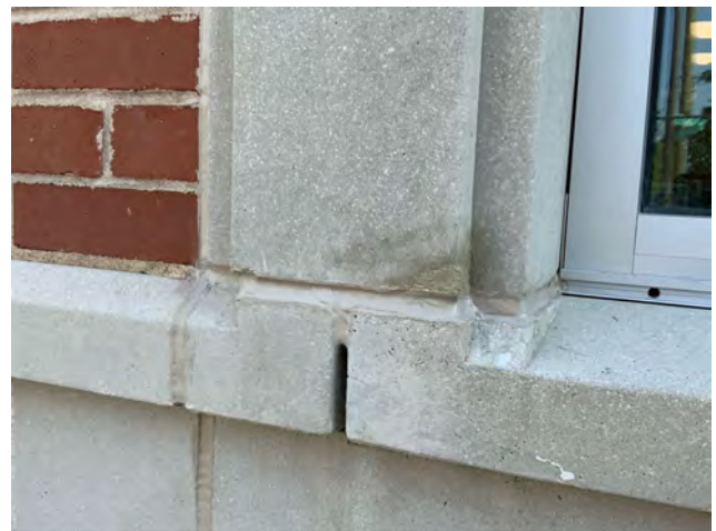
Cast Stone Jamb Repair and Sealant
