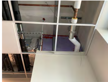
Shaft Wall Construction
