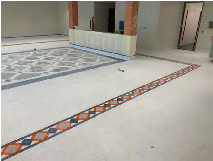
Lobby Terrazzo Flooring
