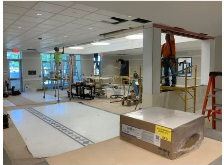
Lobby trim work
