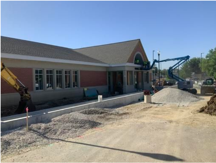
Backfill and site grading
