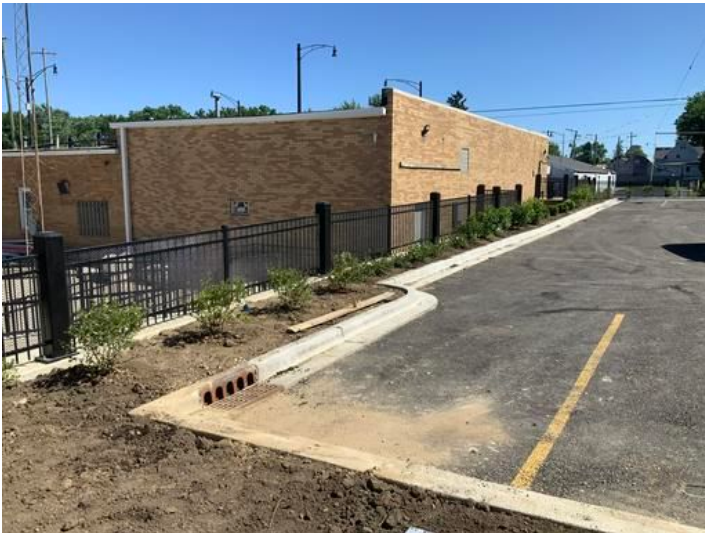
South parking lot landscaping
