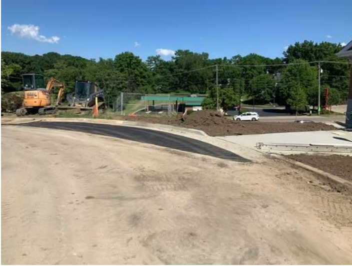
SW corner of site
