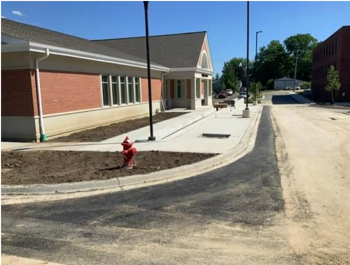
NW corner of site
