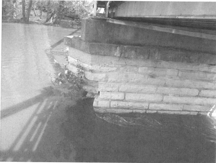
Photo 9 - Northwest Side of West Pier
