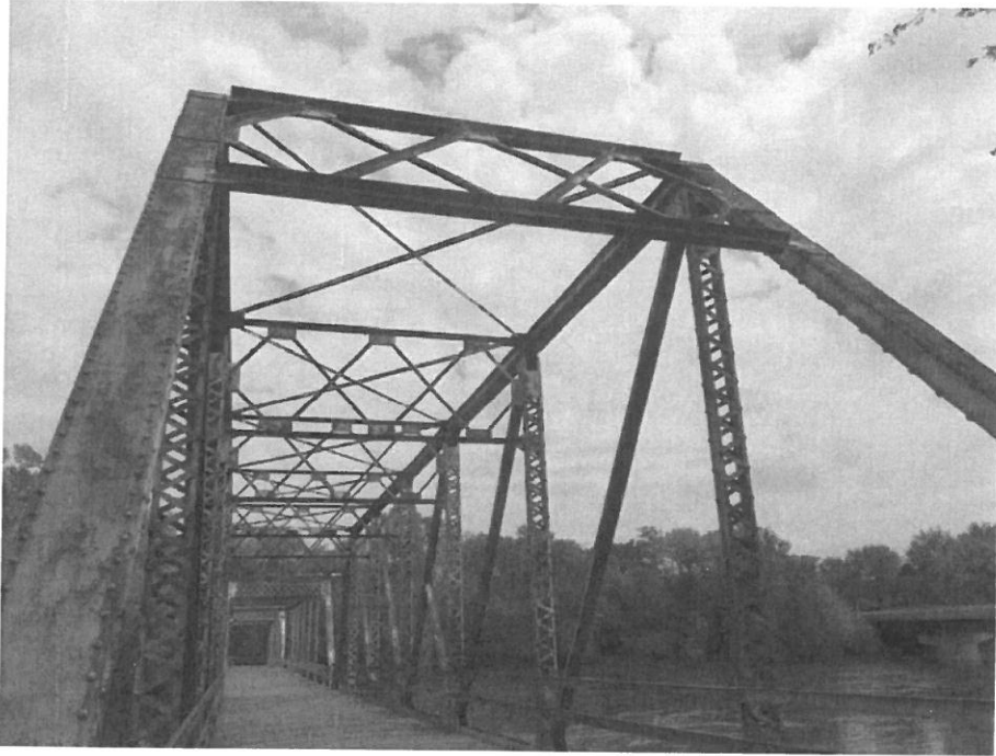
Photo 3 - Looking East at West End of West Truss
