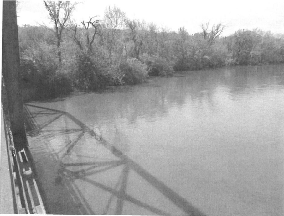
Photo 5 - Northwest from Center of Bridge
