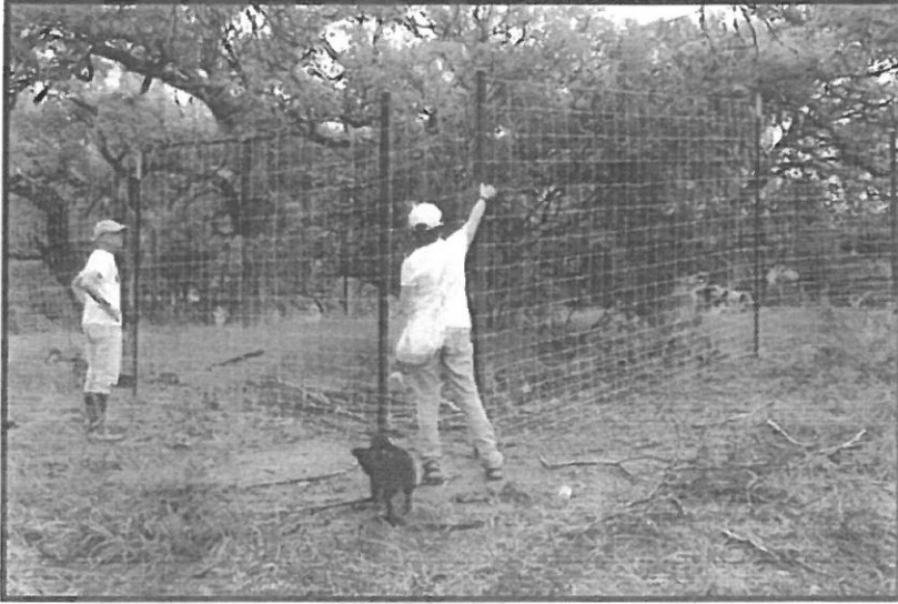
Sample of temporary Corral Fencing:
