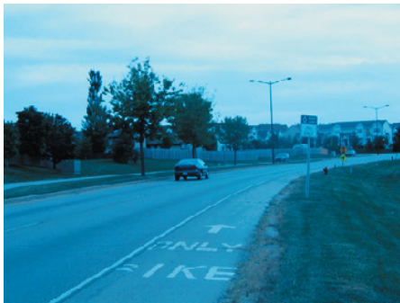
A dedicated bike lane provides a safe path for bicyclists to travel along an urban roadway.
