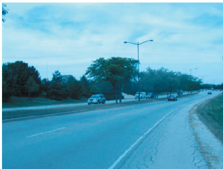
A landscaped median provides an attractive separation between travel lanes on an urban roadway.
